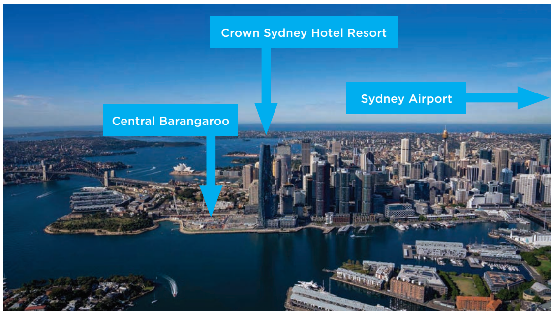
Figure 5: Elevation view image showing existing structures at Barangaroo including the Crown Sydney Hotel Resort. Image credit: Infrastructure NSW, June 2021
