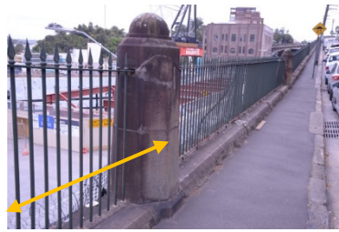
Figure 8.3 Palisade Fence at the central low point of High Street, one of two sandstone piers where the metal bridge to the wharves originally connected to High Street. This opening has been infilled, as shown by the orange arrow. (Source: GML 2020)
