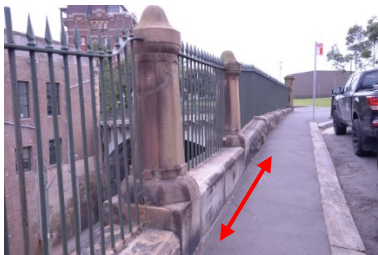
Figure 8.2 Palisade Fence and sandstone piers at High Steps, northern end. The base plinth and fence were infilled (as shown by the red arrow) when the upper stair run was removed. (Source: GML 2020)
