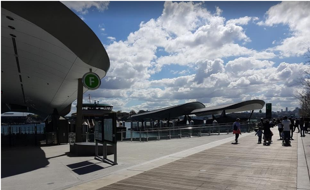
Figure 23 Barangaroo ferry wharf
