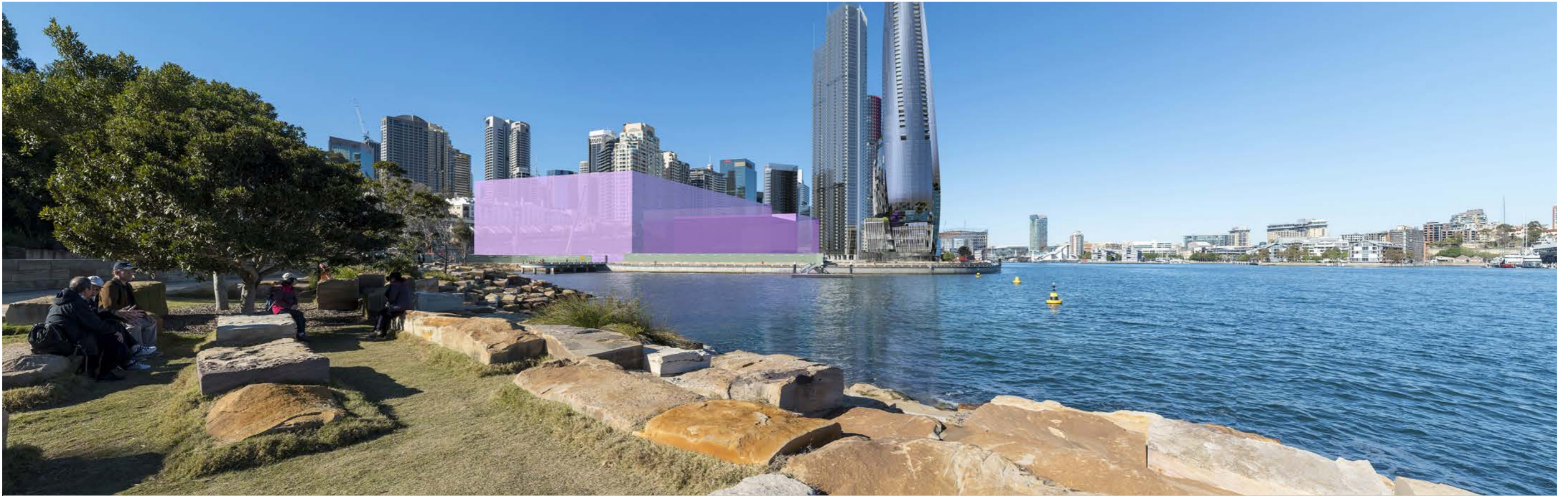
Figure 61 Image showing the development envelope of the Approved Concept Plan (Source: AECOM, July 2018)
