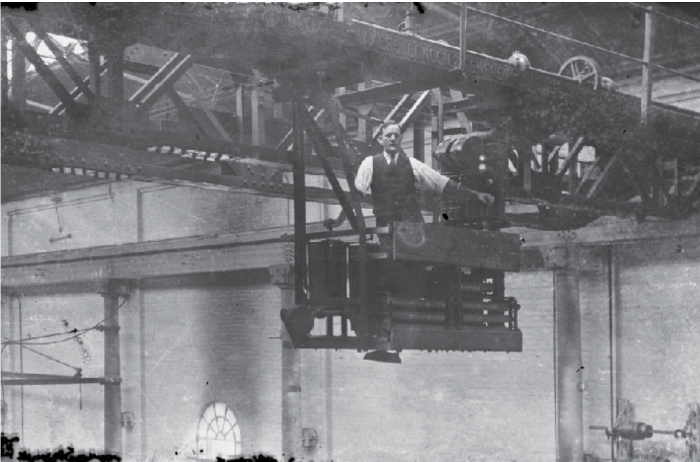
/ Photograph of gantry crane in use with driver in cabin
