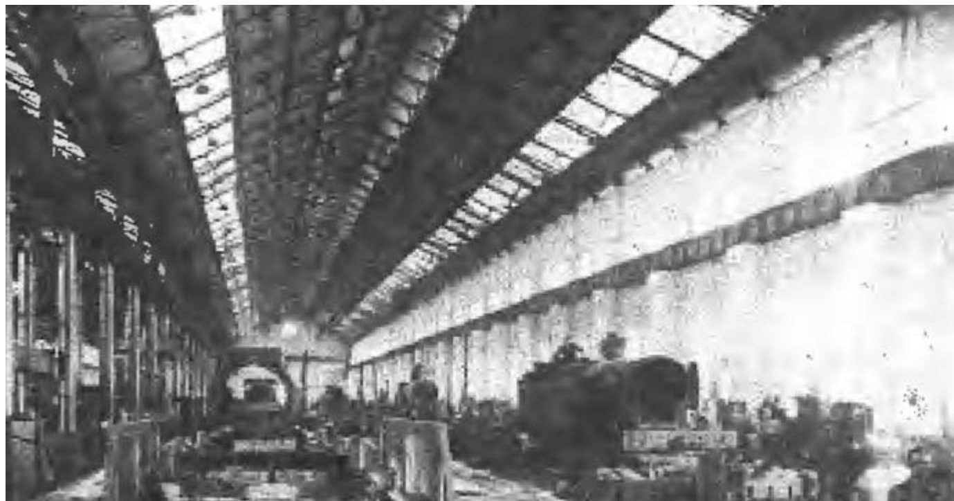
/ Original Arrangement of skylight aligned to main linear axis
