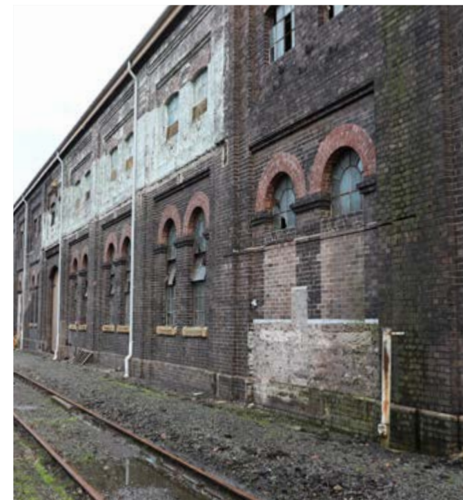
/ Photograph: Existing window openings infilled
