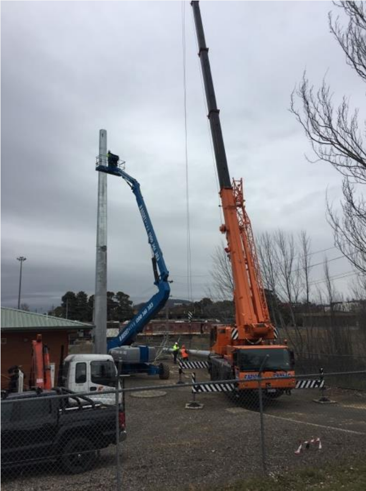
Figure 6-2 | A crane and an elevated work platform assembling a mobile tower
