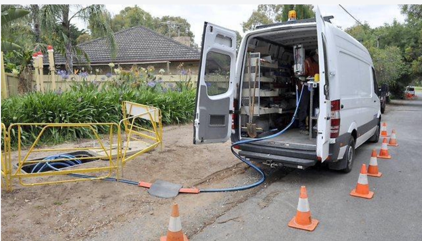
Figure 6-4 | Splicing Van Accessing a roadside pit
