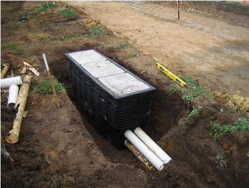
Figure 6-3 | "9 Pit" with multiple P100 conduits being installed
