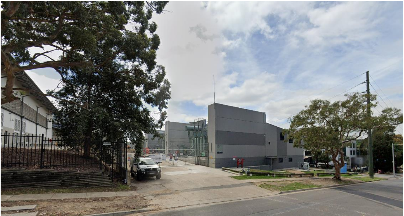
Figure 7: Existing Ausgrid Zone Substation ZN08000 Macquarie Park
