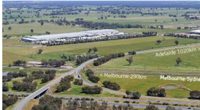
Figure 174. Aerial photo of Logic Precinct
