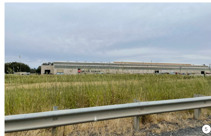
Figure 51. Photograph of Overall Forge. Source: Ethos Urban.
