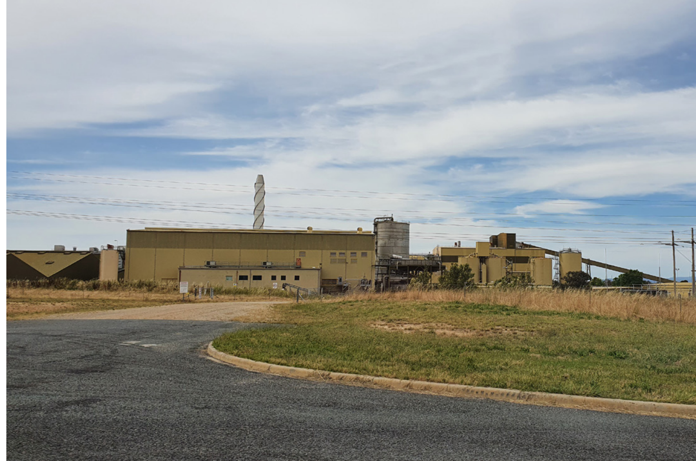
Figure 59. Photograph of the old Paper Mill and disused rail siding. Source: Ethos Urban.
