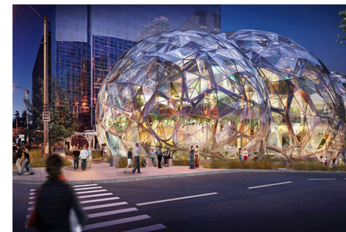
Figure 1.78 Amazon HQ (Source: South Lake Union)
