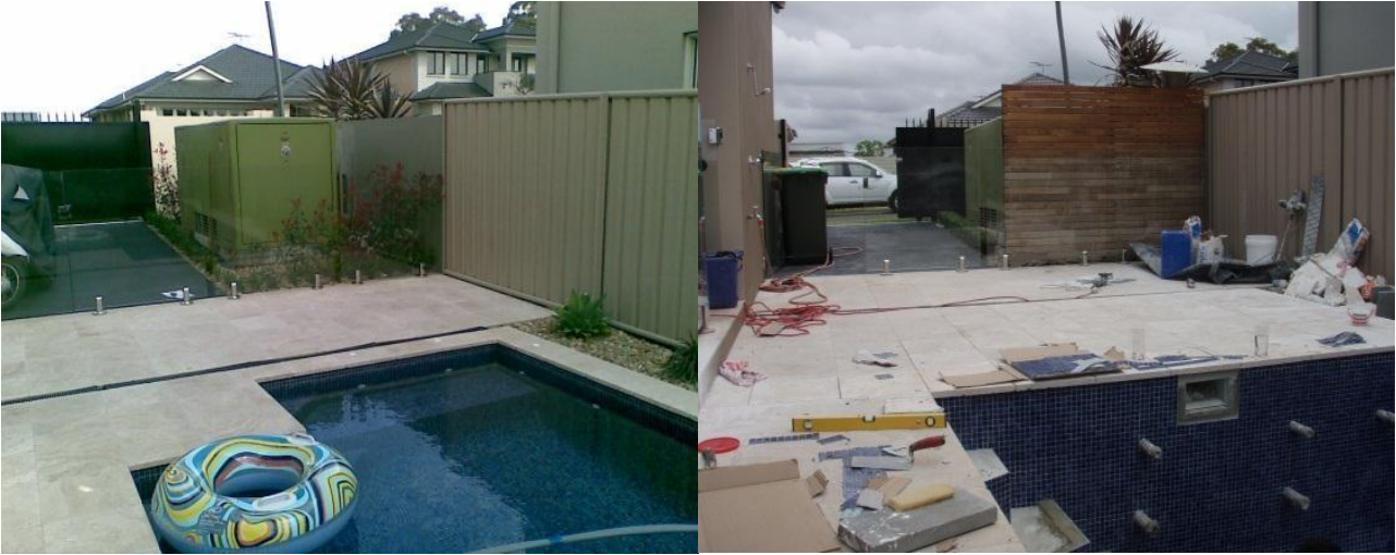
Before and After. This swimming pool in Endeavour Energy's network area at Middleton Grange NSW had to be modified to comply with the restriction for the padmount substation on the use of land in relation to swimming pools.
