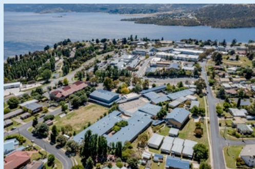
Aerial over existing Jindabyne Central School
