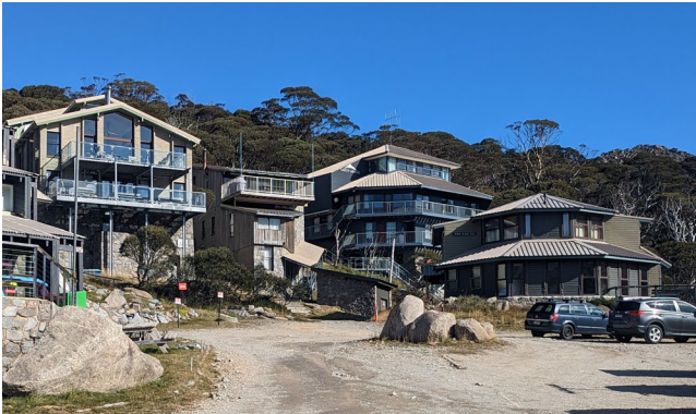
Figure 58. Existing buildings at the end of Charlotte Way
