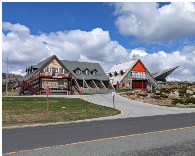
Figure 12. Fire and rescue buildings
