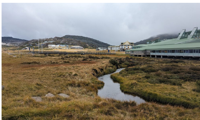
Figure 6. Perisher Centre and creek
