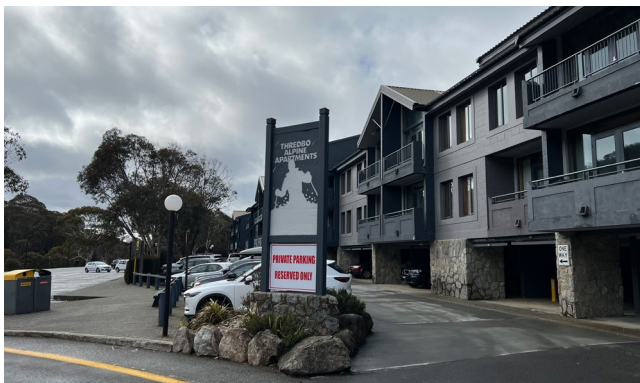
Figure 40. Thredbo Alpine Apartments
