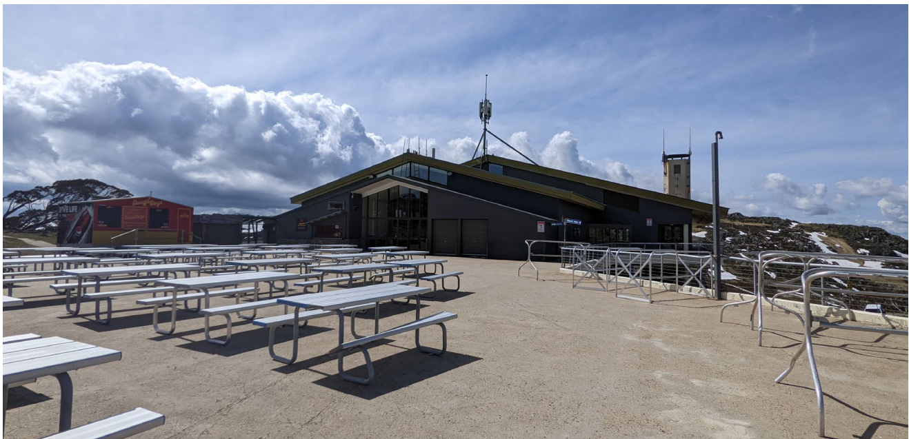
Figure 38. Blue Cow Terminal (south elevation)
