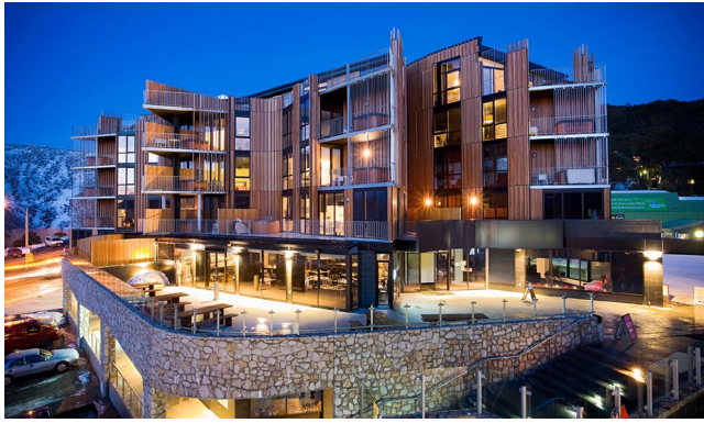
Figure 15. Elevated public plaza with active frontages. Falls Creek, Victoria
