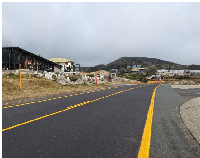
Figure 11. View along Kosciuszko Road (looking south-west)
