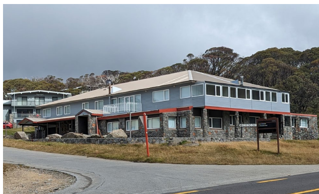
Figure 24. Corroboree Ski Lodge
