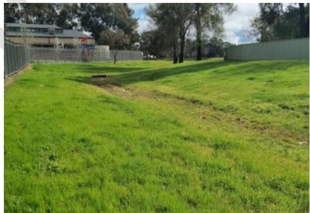
Plate 17 Stormwater drainage line
