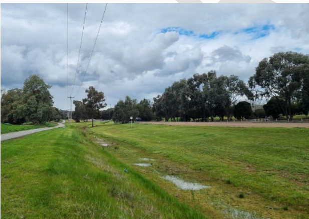
Plate 16 Red Hill Road table drain
