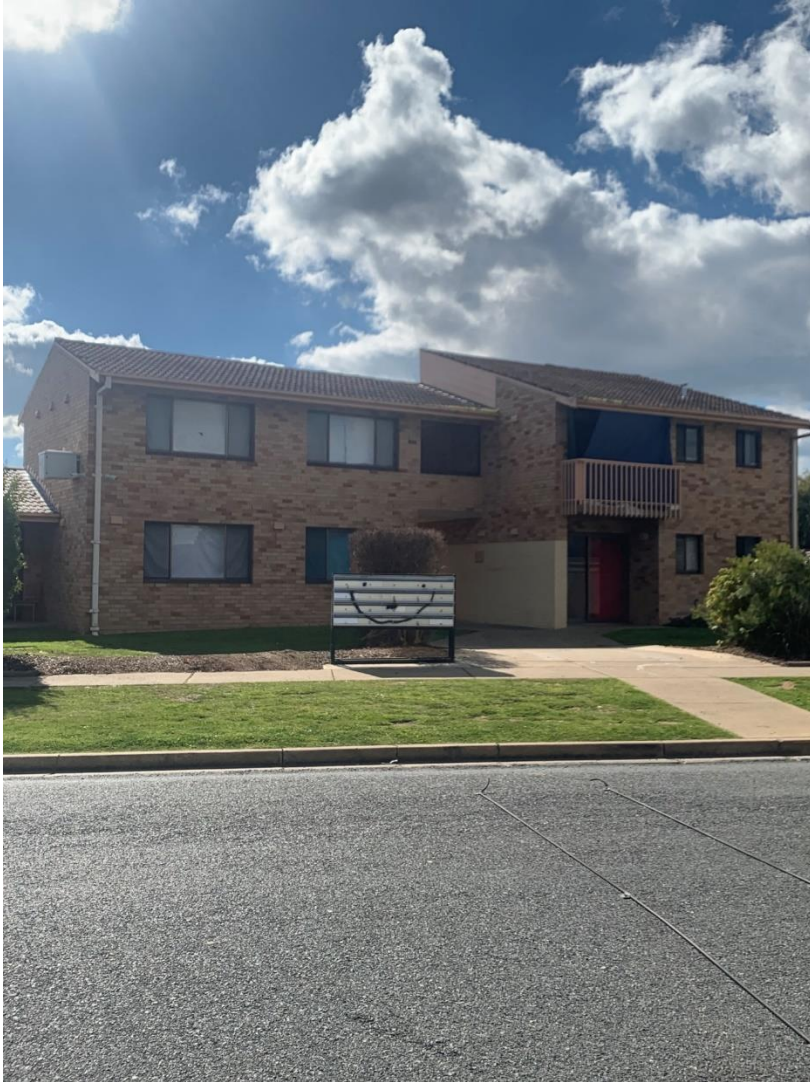
Photograph 5: Typical unit block in Tolland
