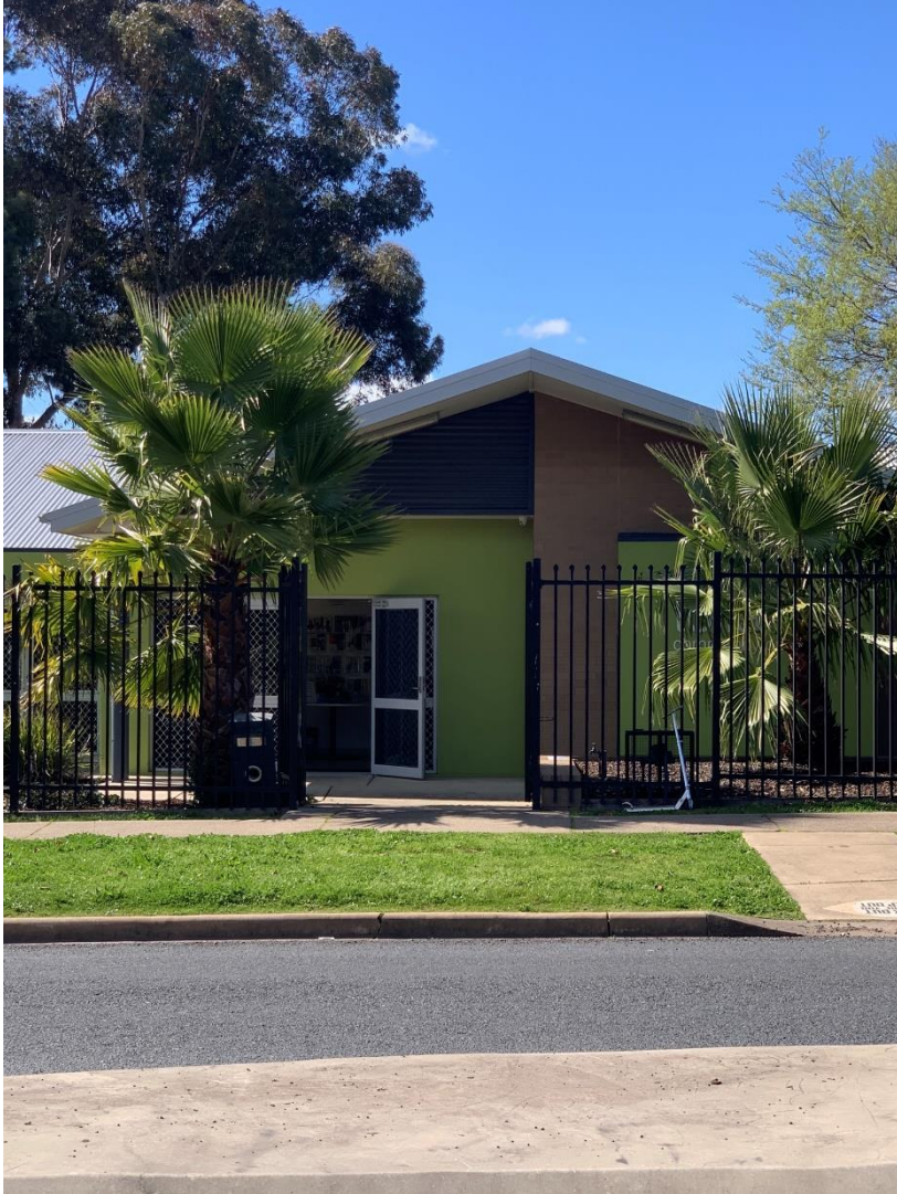
Photograph 7: Tolland Community Centre in Bruce Street
