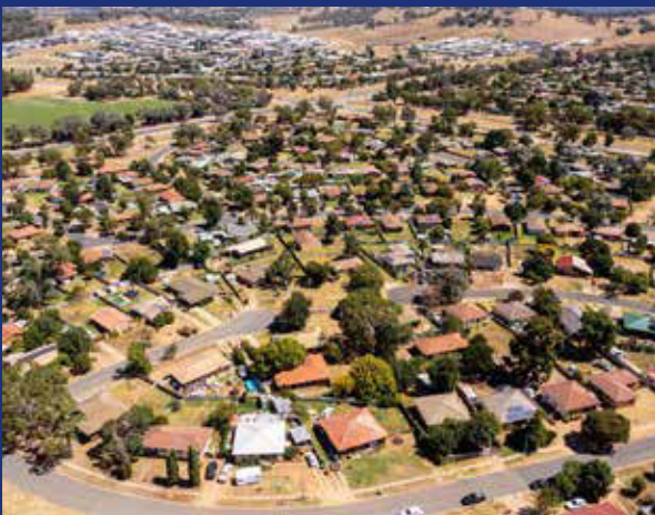
Aerial image, Tolland estate
