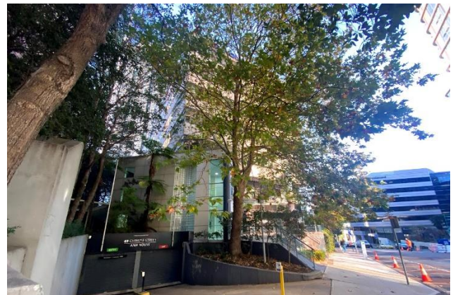
Figure 17 AMA House to the south of the site
