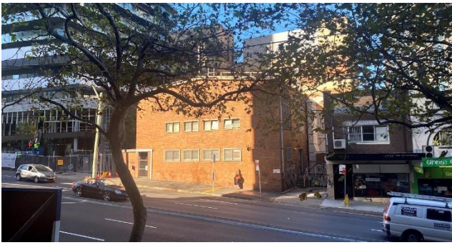
Figure 10 Existing Telstra Exchange Building from Pacific Highway to the north
