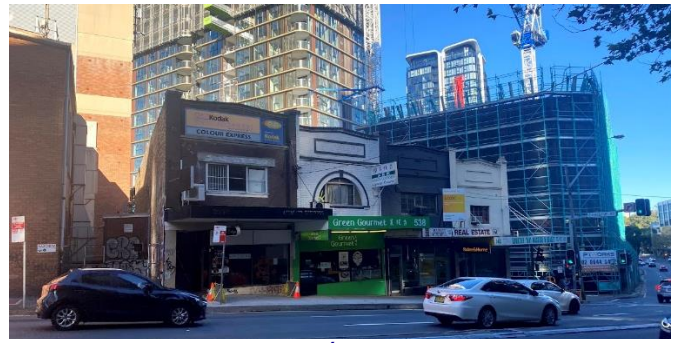
Figure 11 Existing retail/commercial buildings from Pacific Highway to the north
