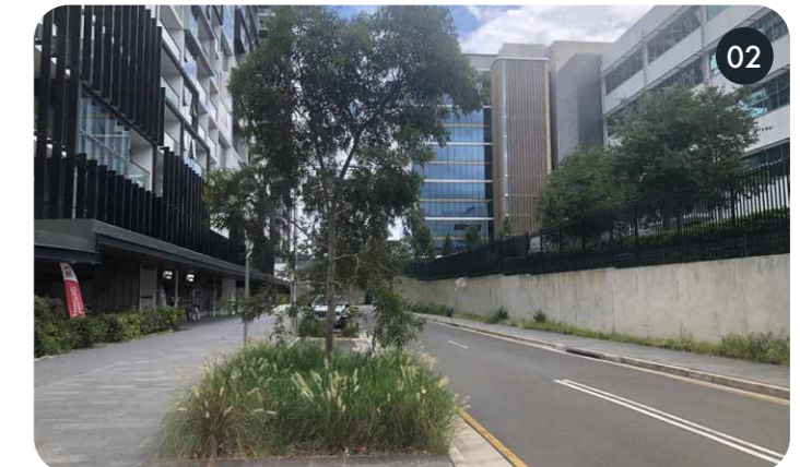
Retaining wall on private lot boundary
