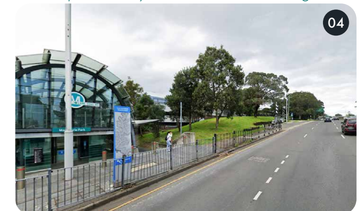
Lane Cove Road level change around Metro
