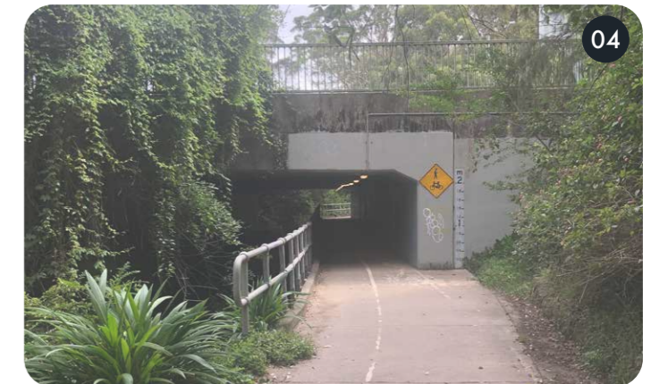
Shared path under Epping Road
