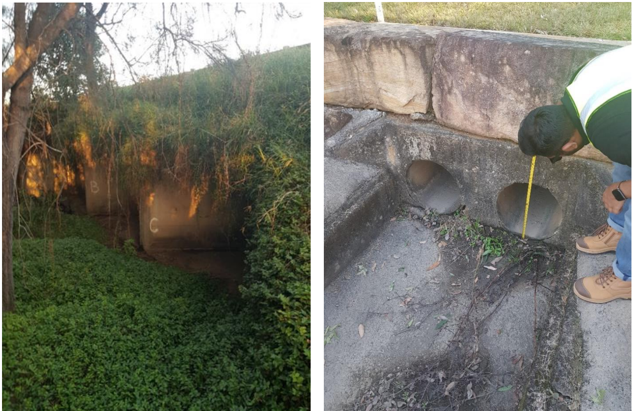
Figure 2-1 Claremont Creek: Culverts Under M4 Motorway (left). Samuel Marsden Drive. Twin Circular Culverts (Right)
