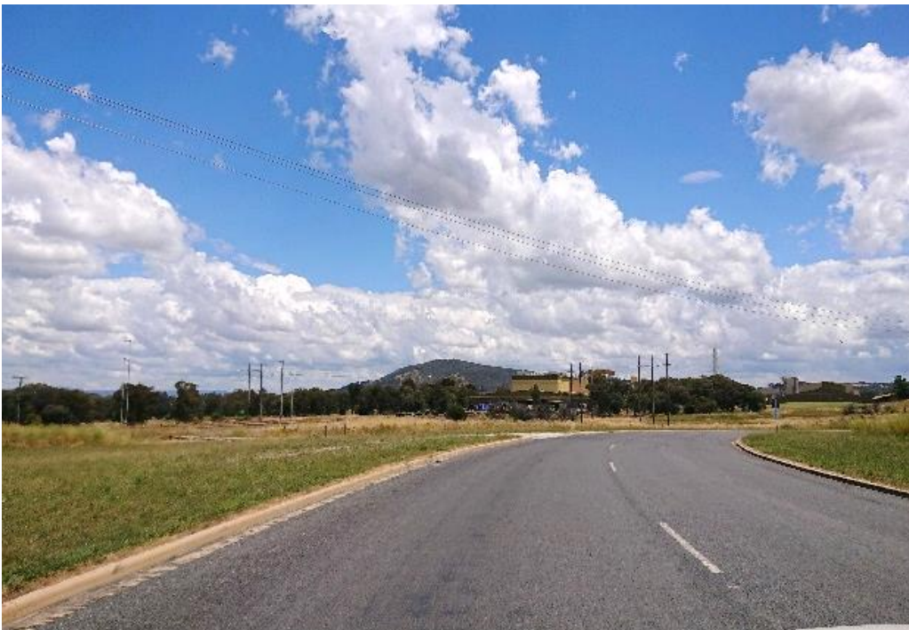
Figure 3-5 | A view looking south-west at the Visy owned site
