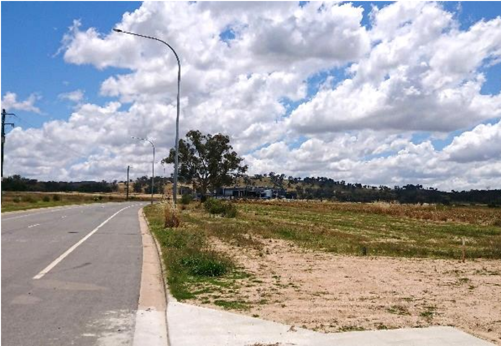
Figure 3-2 | A view looking north at the new Plastic Recycling centre
