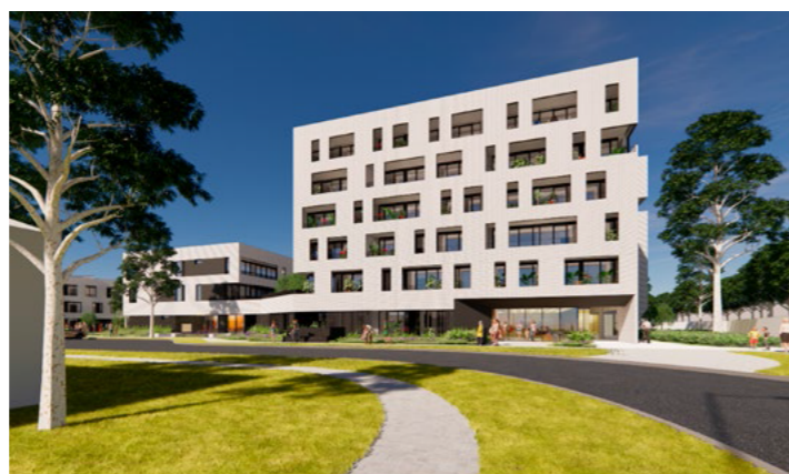
Figure 1.12 View to new apartments (Source: Victoria Homes)
