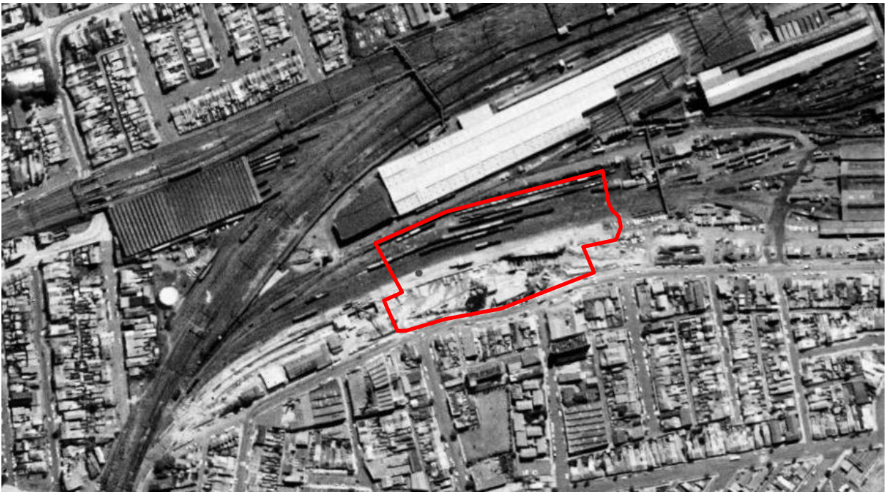
Figure 39 – Aerial photograph from 1975 showing construction works being carried out within the subject site. The subject site is overlaid.
