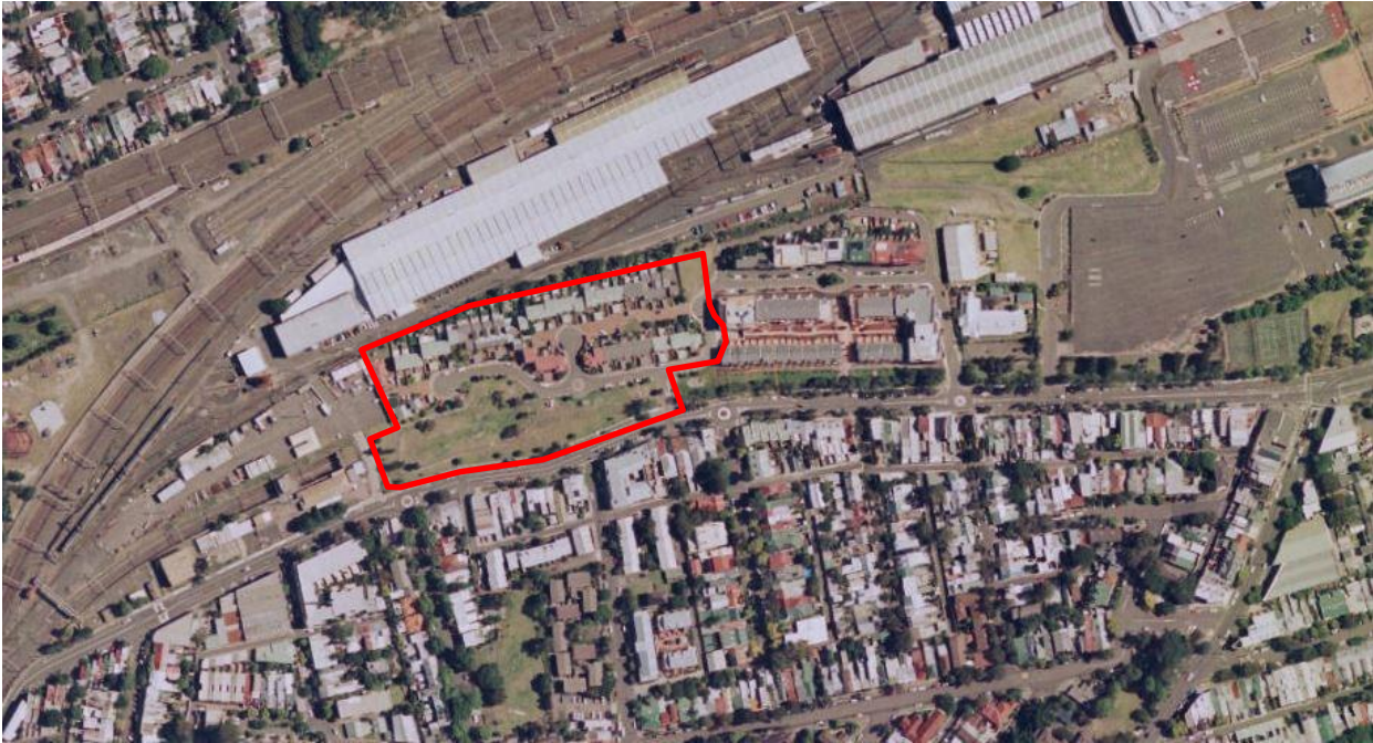
Figure 42 – Aerial photograph from 2005 showing the Explorer Street social housing site. The subject site is overlaid.
