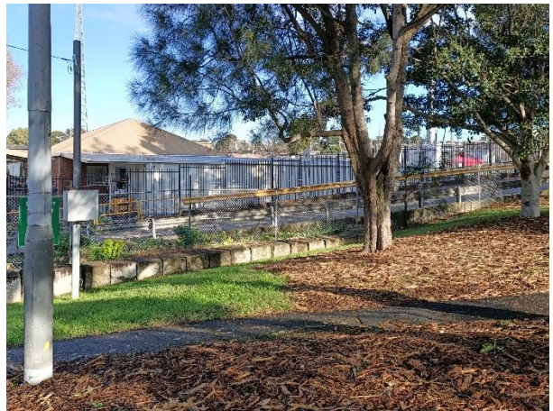
Figure 31 – Western end of South Sydney Rotary Park showing boundary with New Inner City Fleet Eveleigh Facility.
