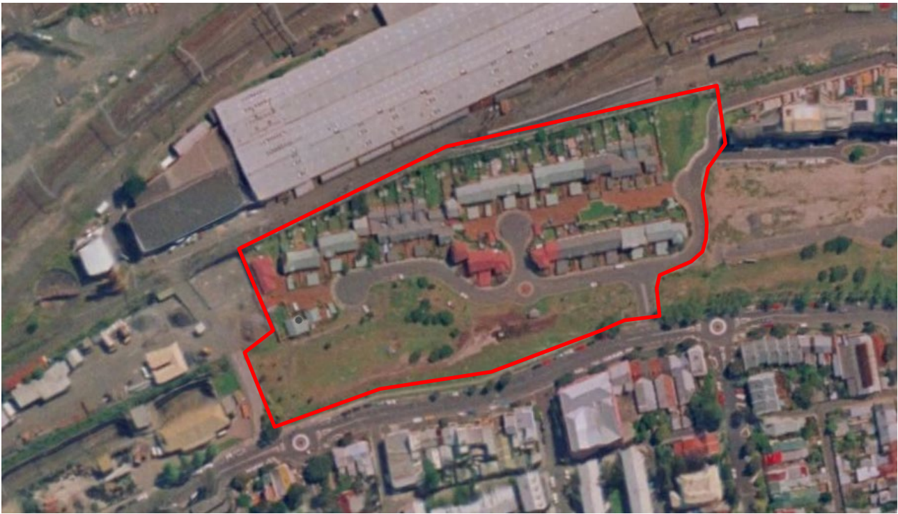
Figure 14 – 1998 aerial photograph indicating that the subject area had been resumed for social housing purposes by this date.
