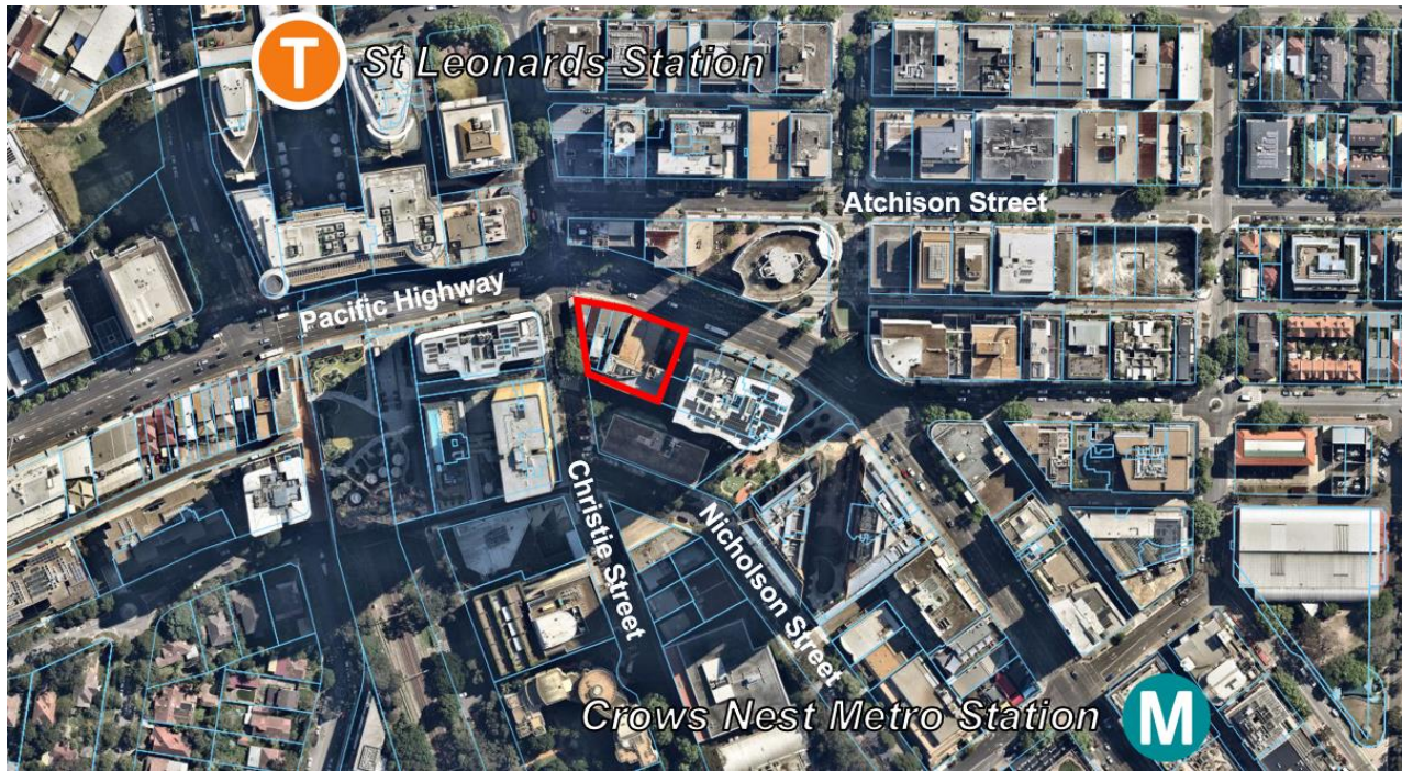
Figure 1: St Leonards Telstra Exchange Site (524-542 Pacific Highway, St Leonards) location and context (Nearmap).
