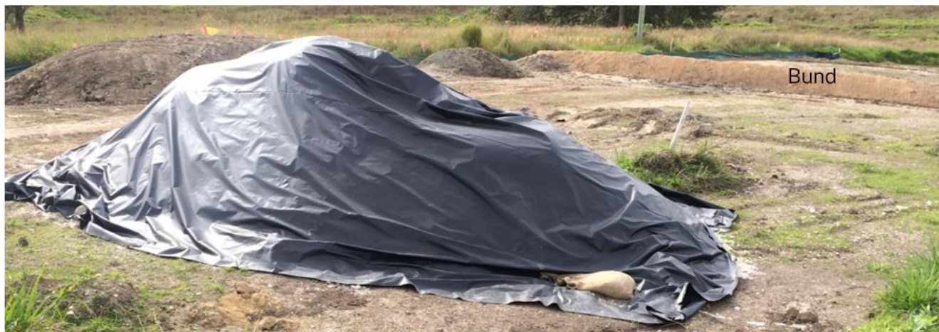
Figure 7. An unattended stockpile has been securely covered to prevent any loss of soil, with a compacted bund acting as sediment control downslope. Source: Department of Primary Industries – Fisheries
