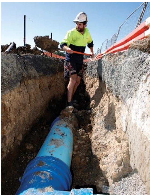
Figure 13. A construction worker installs a service trench
