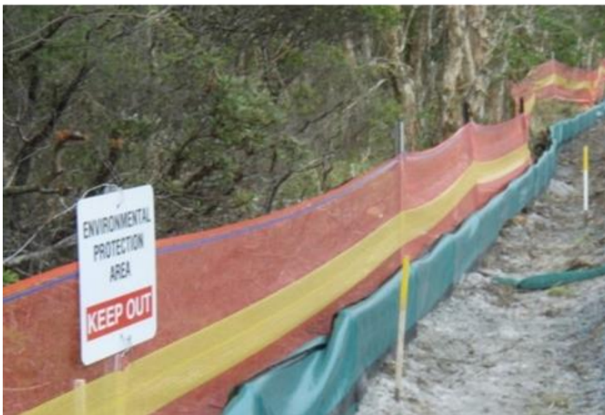
Figure 3. A no-go area on a construction site. Source: Department of Primary Industries – Fisheries
