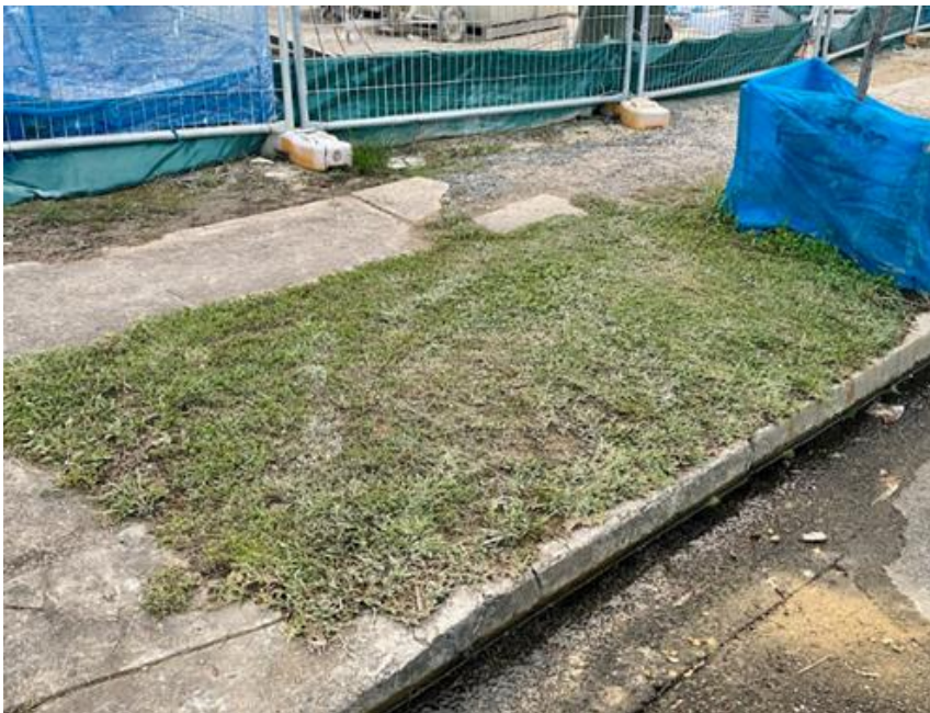
Figure 11. Grass strips by a road that control sediment in low flows. Source: Parramatta River Catchment Group
