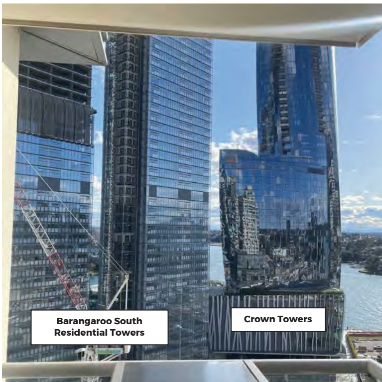
Photo 1: Obstructed views from balcony of Apartment No. 1506 (Level 15), view west Source: Milestone, 2022
