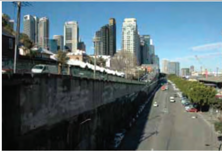
Figure 4 View north-east from the Munn Street bridge of Hickson Street and the High Street cutting. The slope falls away to a dip and rises again to the south seems to mark the pattern of quarrying (City Plan Heritage, 2006, p. 61)
