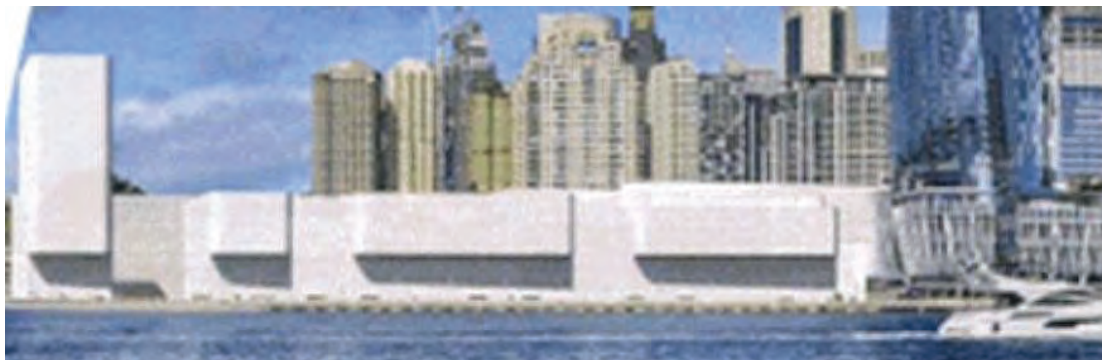
1The new height adversely impact the image to the indigenous space, damage the serenity of a heritage site, loss of view to residents and visitors to the Observatory Hill
