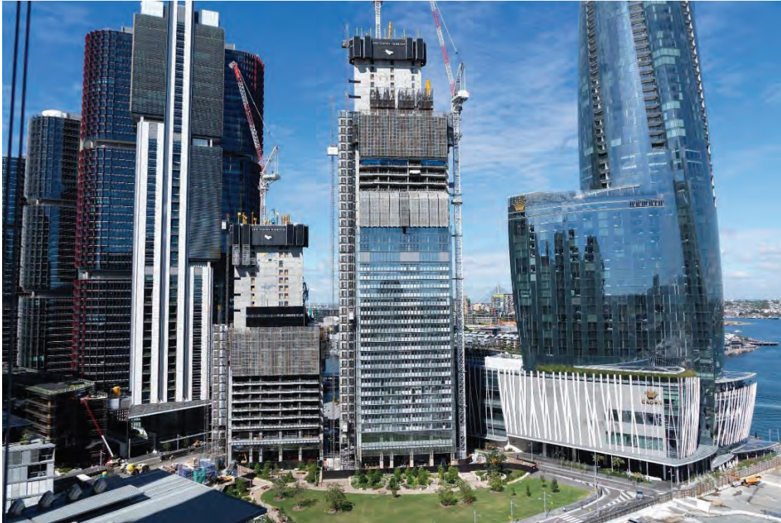
Figure 68 Current view from mid-level northwest corner of Highgate
