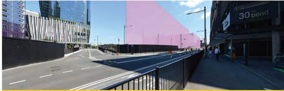
Figure 71 Image showing the development envelope of the proposed Hickson Road. (Source: AECOM, February 2021)
