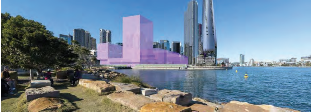
Figure 7: Proposed Concept Plan under MOD 9, view southeast from Barangaroo Reserve Source: AECOM, 2021
