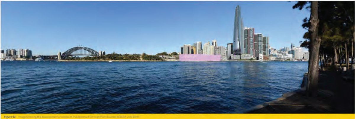
Figure 52 Image showing the development and the proposed bridge from Balmain, NSW, July 2018
