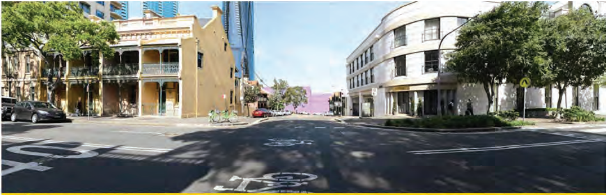
Figure 45: Street showing the development components and building envelope (View 45 from 1/2/2014, February 2014)
