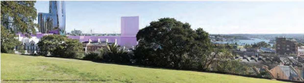
Extract 3: Showing poor layout of Block 7 from Page 89 of the Urban Design Report (Appendix E)
