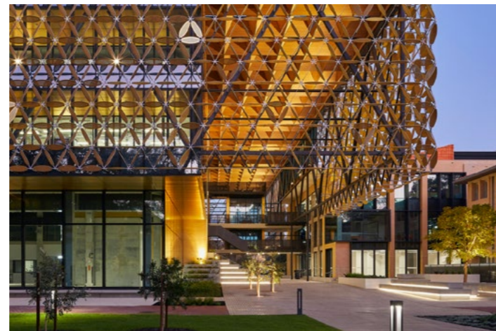
A veil façade with petals fixed at different angles to suit their orientation mitigates glare, heat, and filters sunlight.
