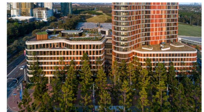
Barangaroo South and Boomerang Tower both show the use of stepped buildings, awnings and trees to mitigate wind impacts.
