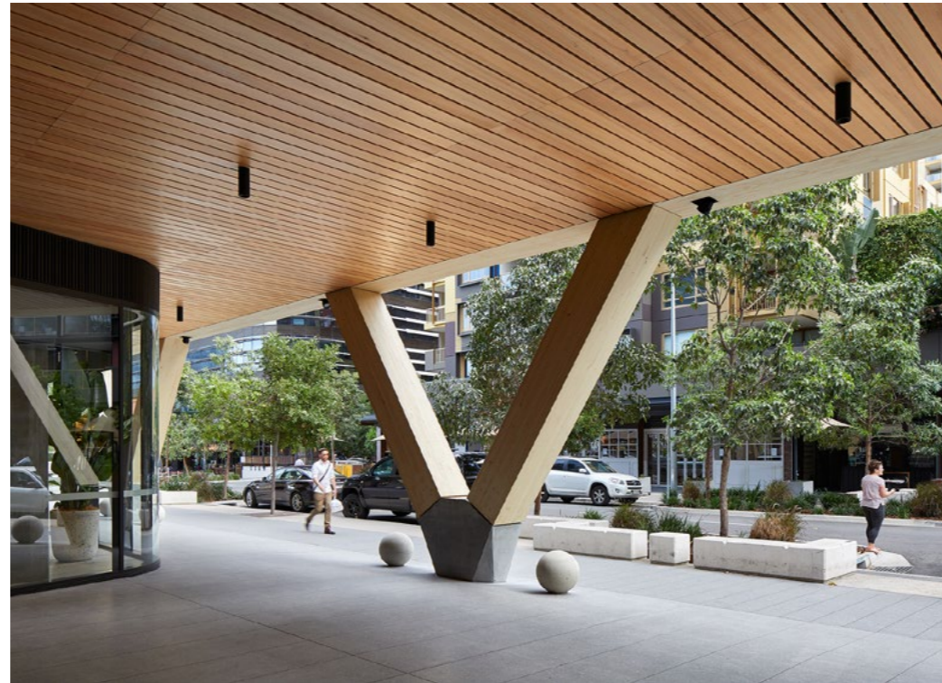
CLT structure. King Street, Brisbane.
