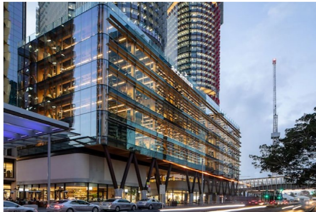
Material selection to reduce reflectivity to the public domain International House, Barangaroo
