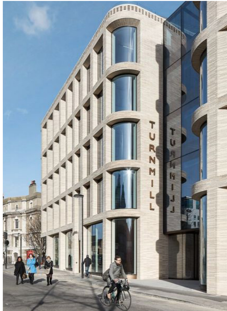
Turmill, London by Piercy & Company (Source : Hufton+Crow)
