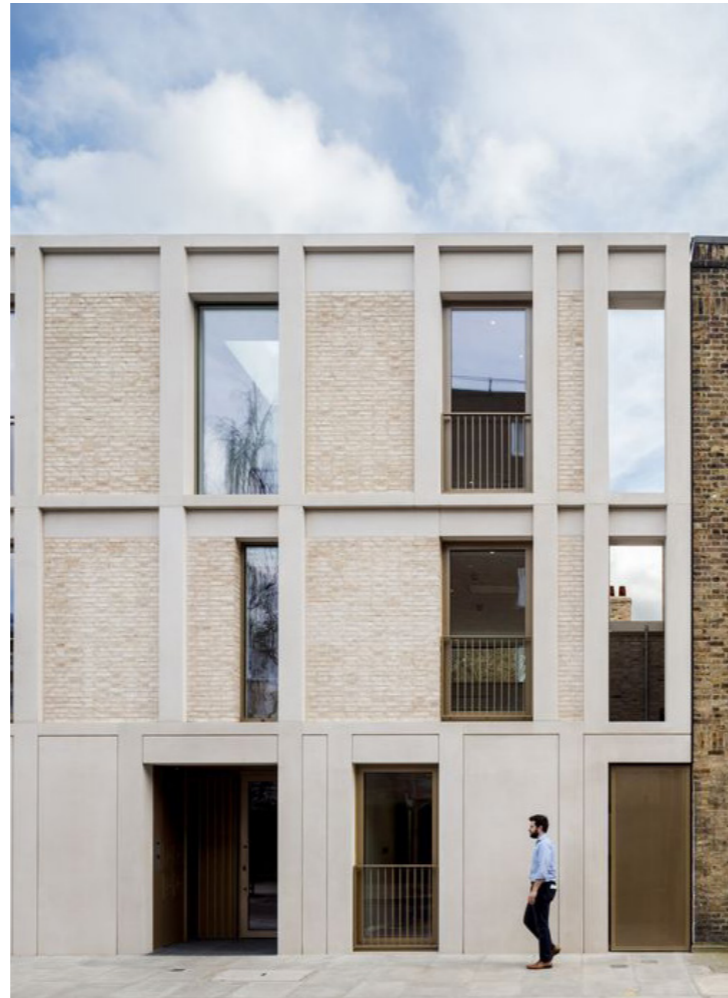
Residential building, London by Haptic (Source : Simon Kennedy)
