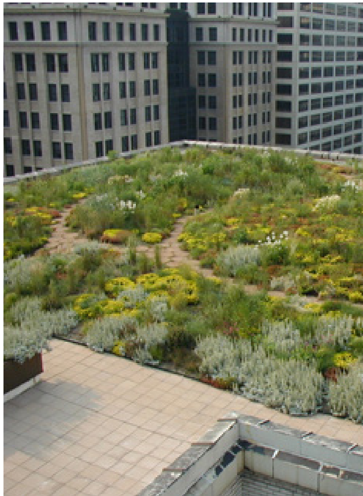
Chicago City Hall Green Roof, Chicago (Source: Inhabitat.com)
