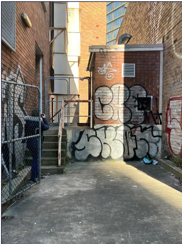
Photograph 12: Void between 524 Pacific Highway and 536 Pacific Highway.
