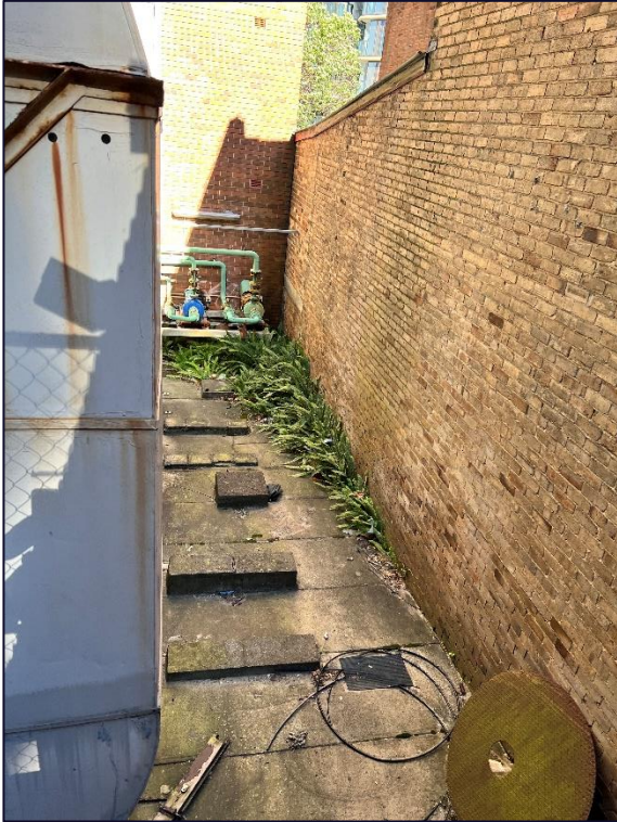
Photograph 13: Area accessible through a vertical ladder between at 524 Pacific Highway and 536 Pacific Highway.
