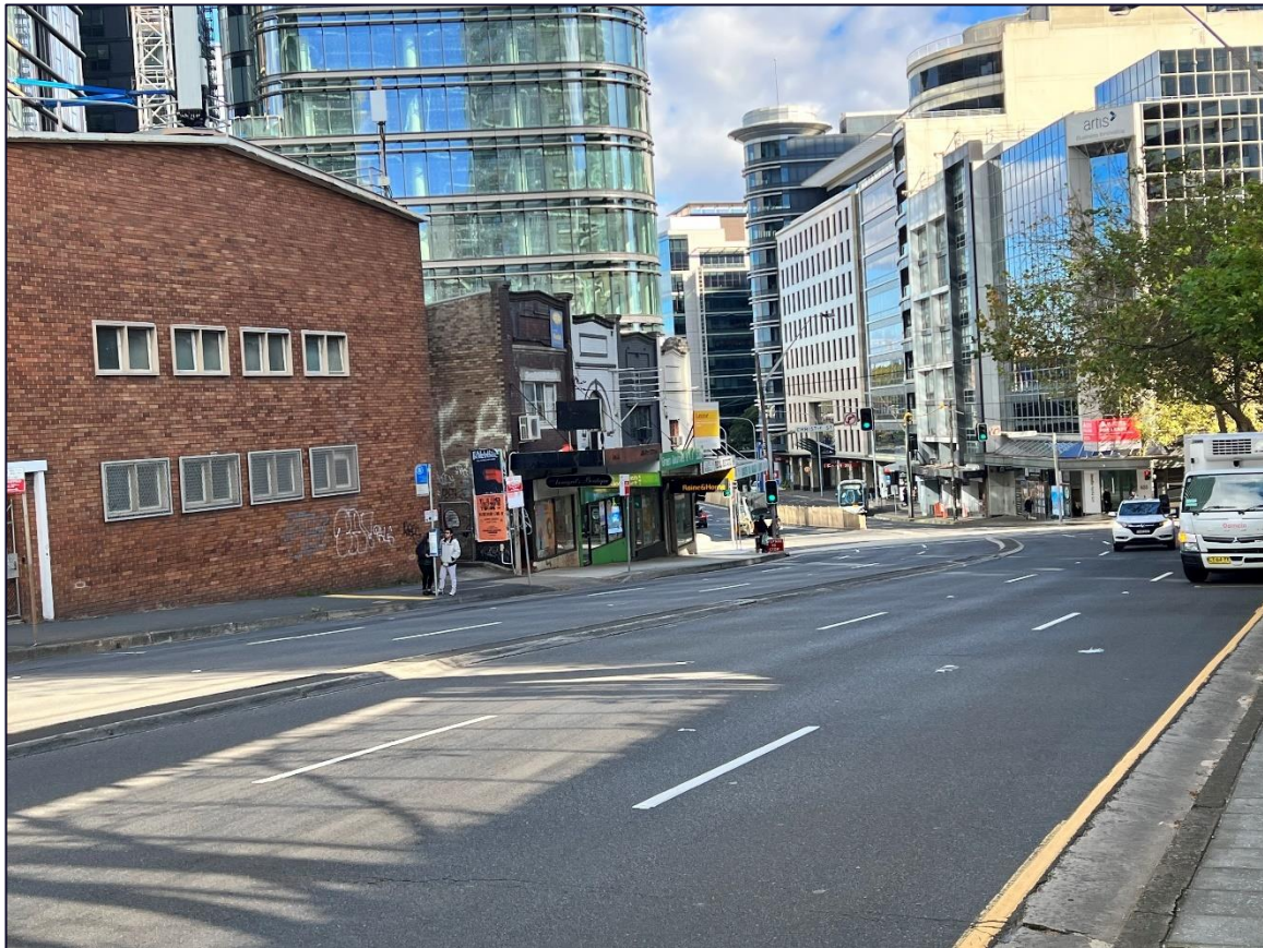
Photograph 2: Photo of the study area showing the Pacific Highway sloping down towards Christie St. This building contains a basement and underground services
