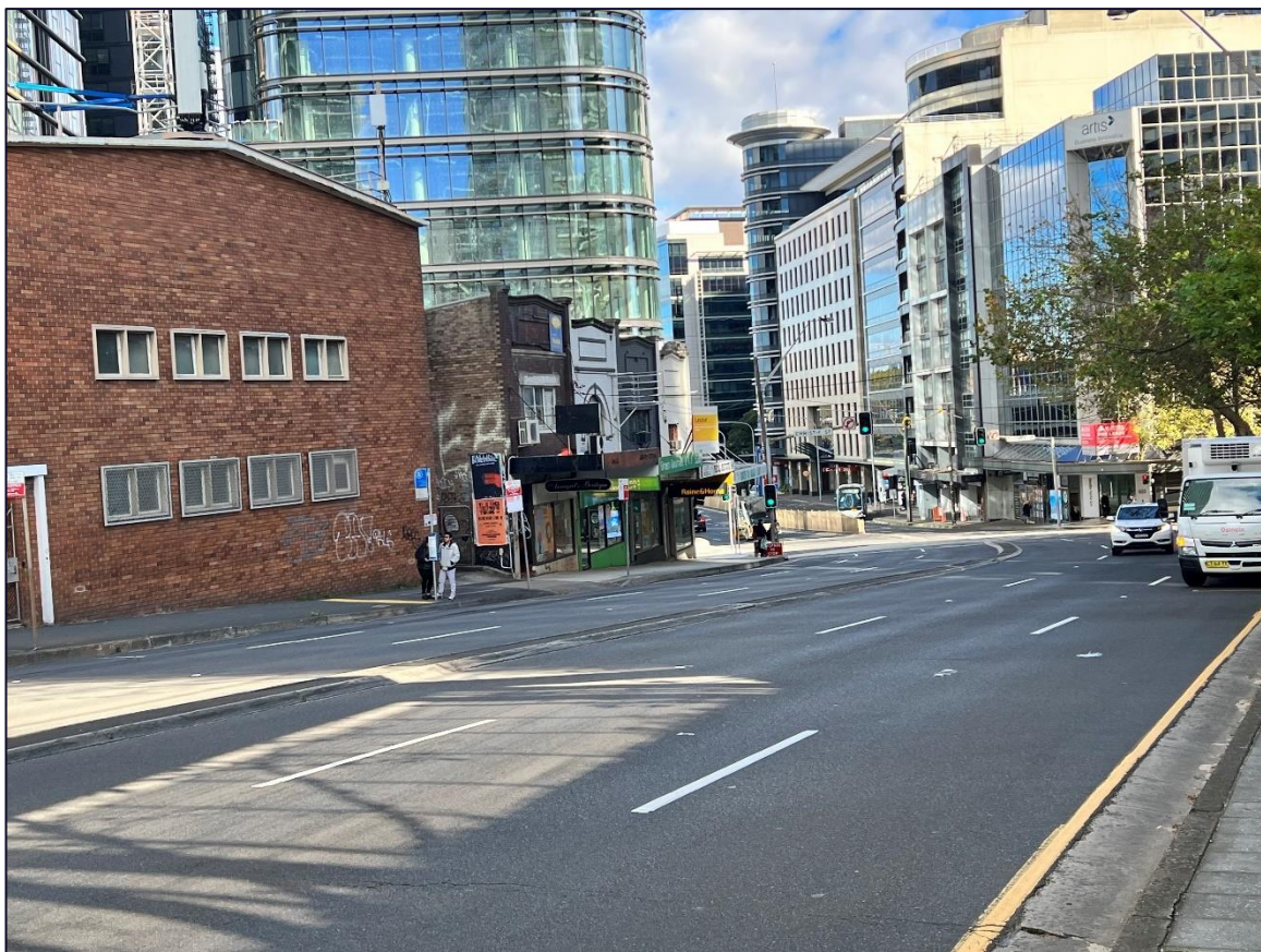
Photograph 2: Photo of the study area showing the Pacific Highway sloping down towards Christie St. This building contains a basement and underground services
