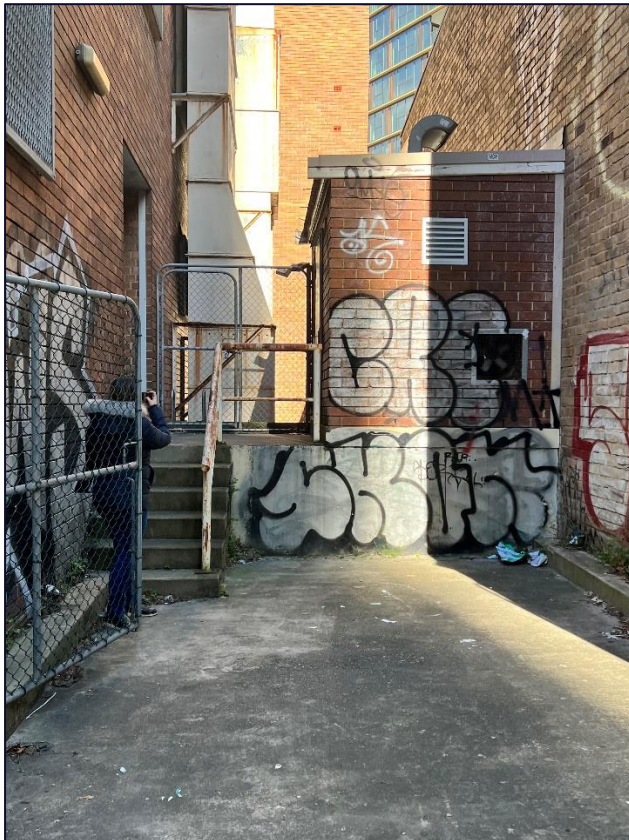
Photograph 12: Void between 524 Pacific Highway and 536 Pacific Highway.
