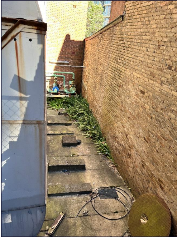
Photograph 13: Area accessible through a vertical ladder between at 524 Pacific Highway and 536 Pacific Highway.
