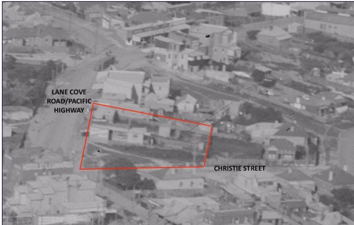
Figure 12: Part of an undated (c.1930-32) aerial photograph of St Leonards providing evidence of buildings on Lots 7, 8 and 9 while Lot 10 remained undeveloped (Milton Kent ON 447/Box 026 Item 02 SLNSW).
