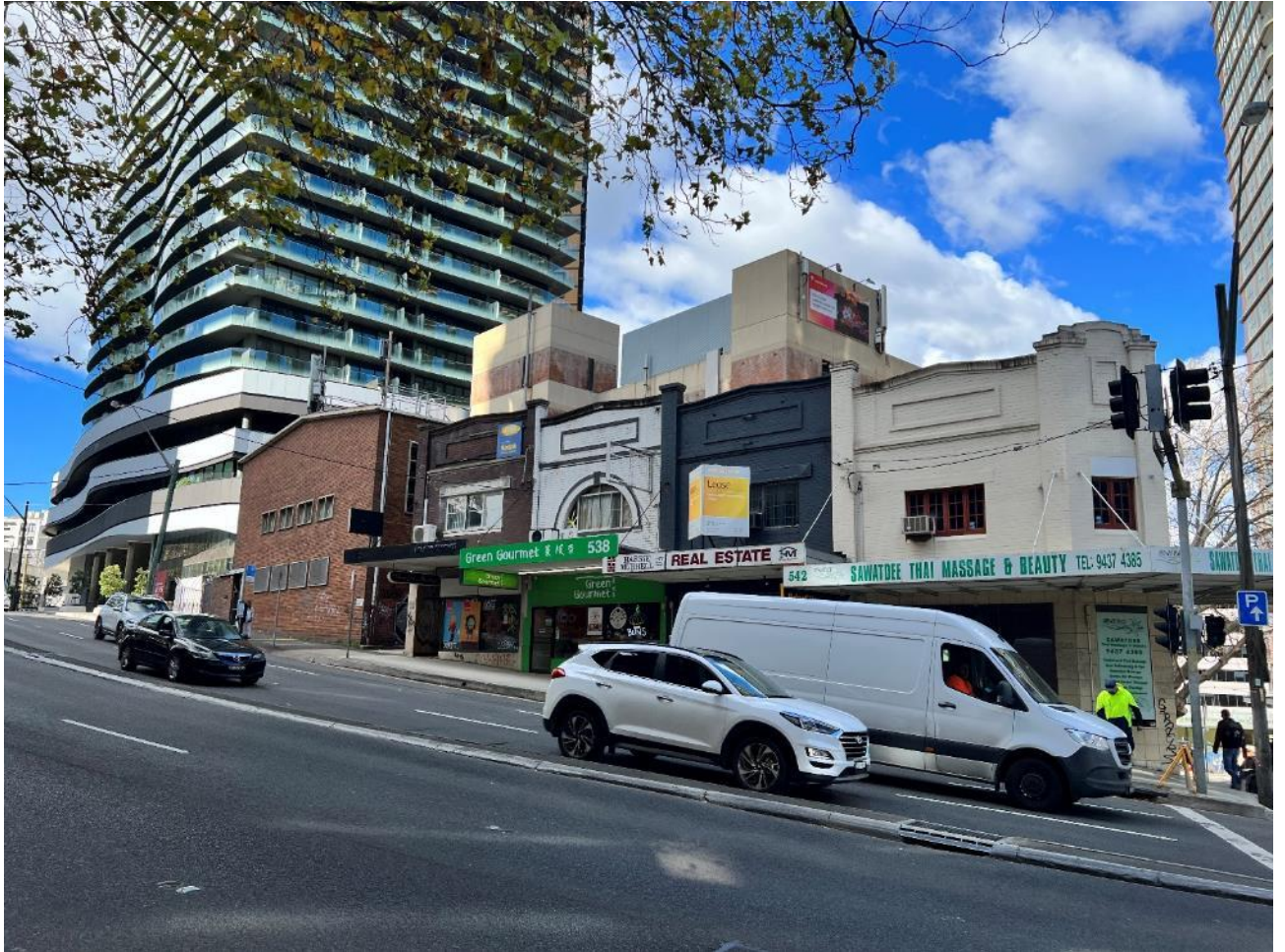
Photograph 1: Study area. Camera facing south east from the corner of the Pacific Highway and Christie Street.
