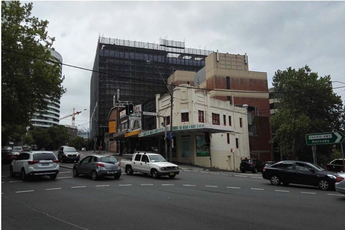
Photograph 1: Site area (looking south-east)
