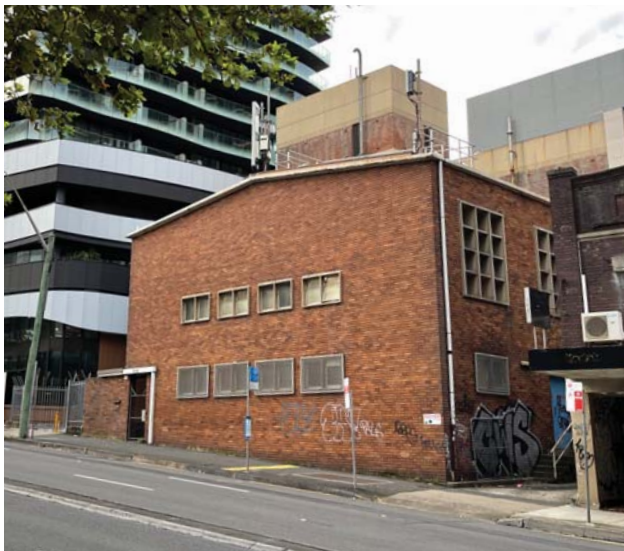
Pacific Highway interface as a three storey structure
