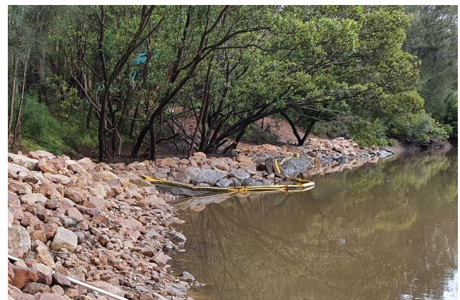
Figure 28. Works completed in 2022 to address unstable banks of Haslams Creek near Kronos Hill
