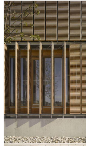
Image: Shade structures and natural materials to keep the heat out when necessary.
