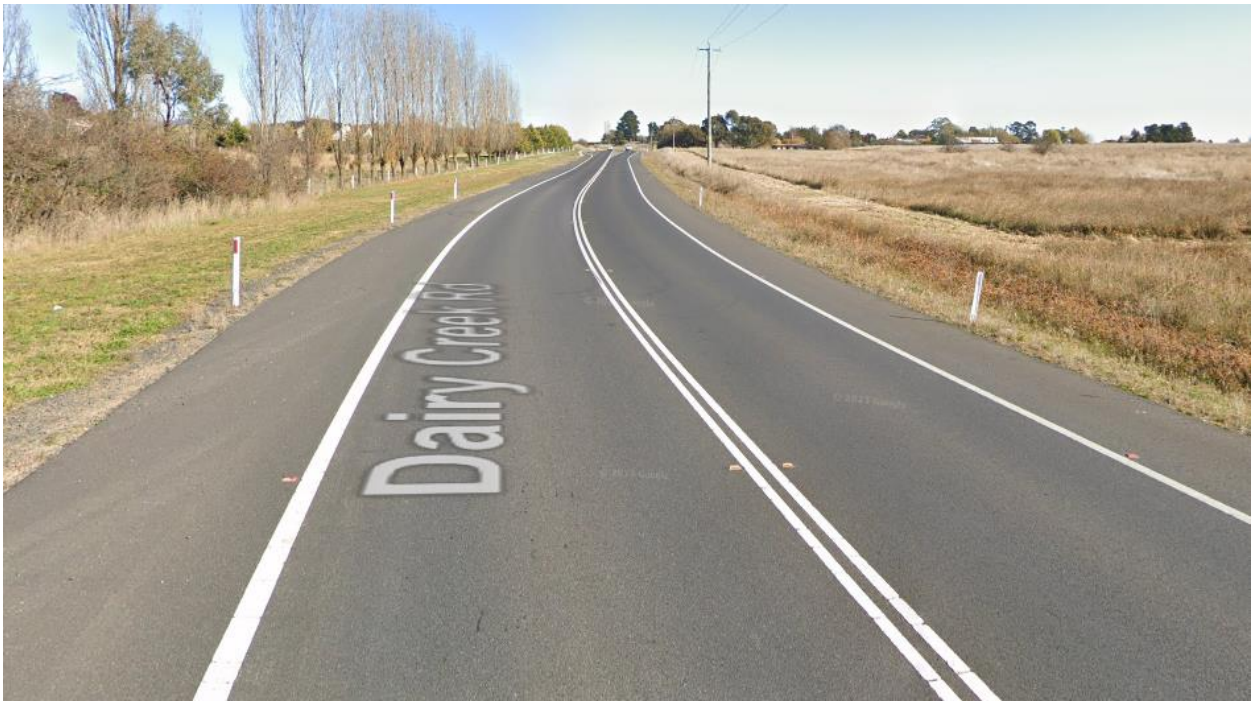
Figure 2.3 Dairy Creek Road in proximity to the Site
