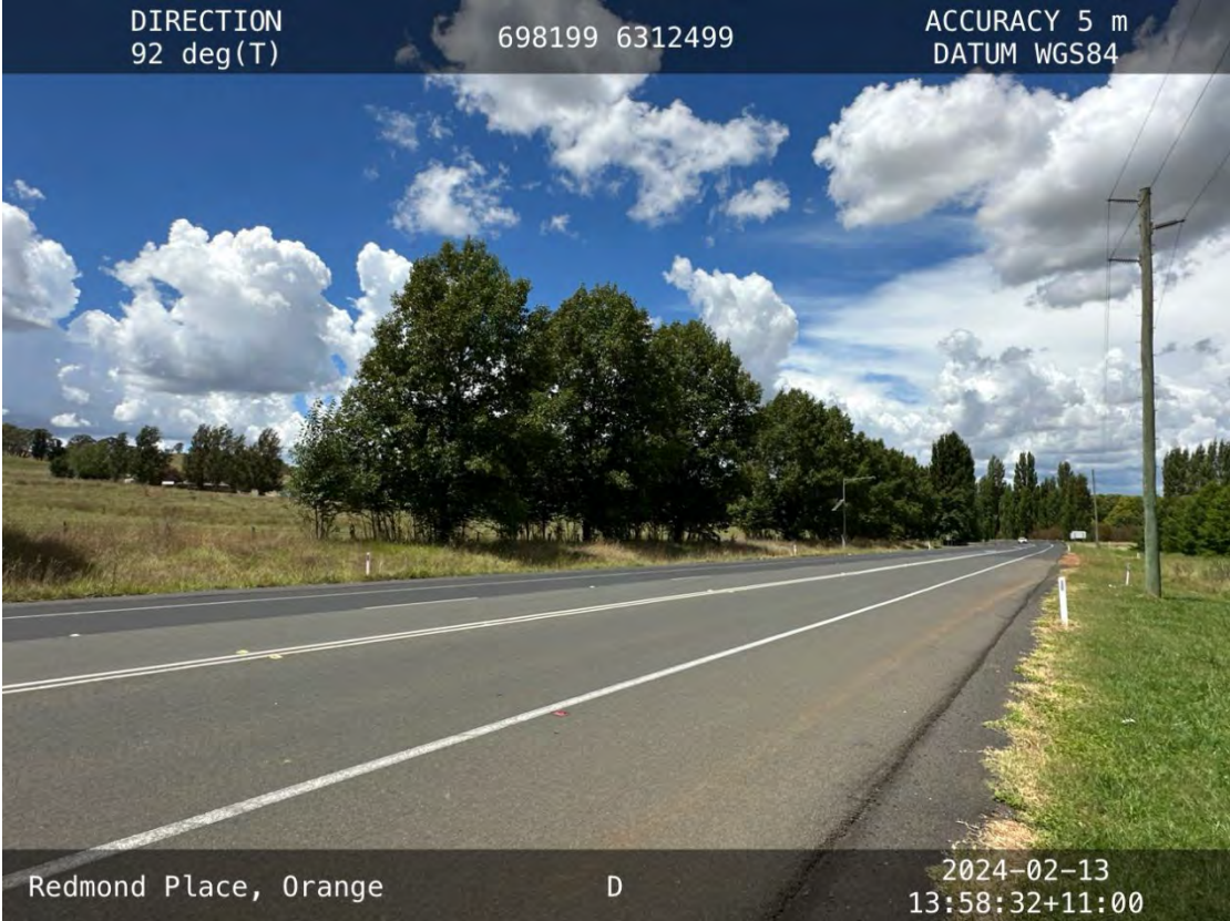
Plate 83: Bathurst Road looking south adjacent to the southern end of the site
