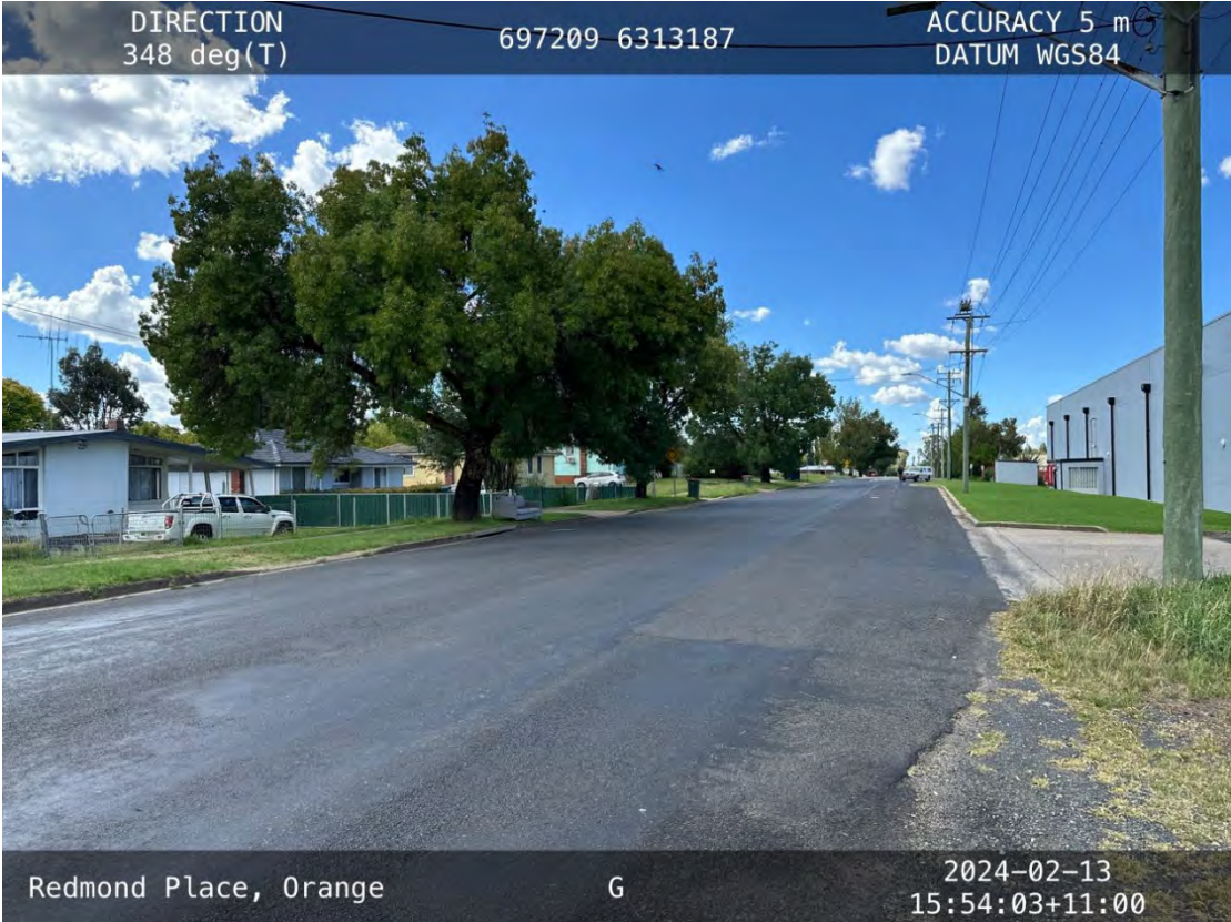
Plate 86: Lone Pine Avenue Looking north from north western corner of site
