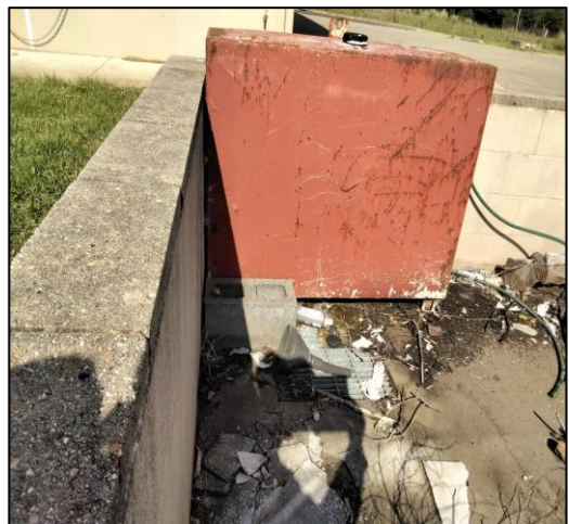
Photo 16 Sump within AST bund facing east (30 January 2024)
