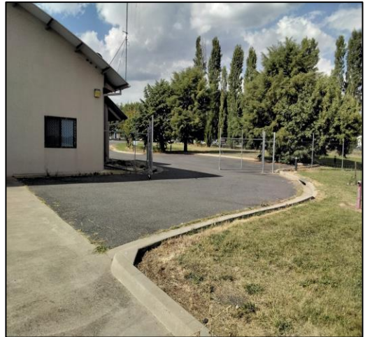
Photo 20 Entry gates to helipad area facing north (30 January 2024)
