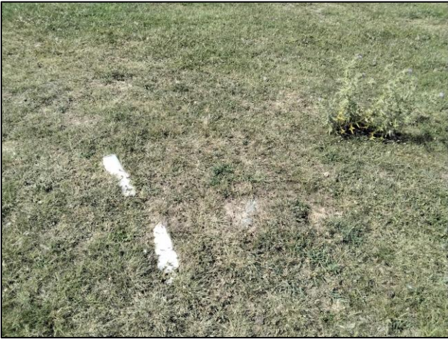
Photo 7 Potential asbestos containing material (cement pipe) Lot 1 (30 January 2024)
