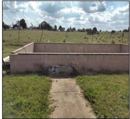
Photo 12 Former AST bund facing west (30 January 2024)
