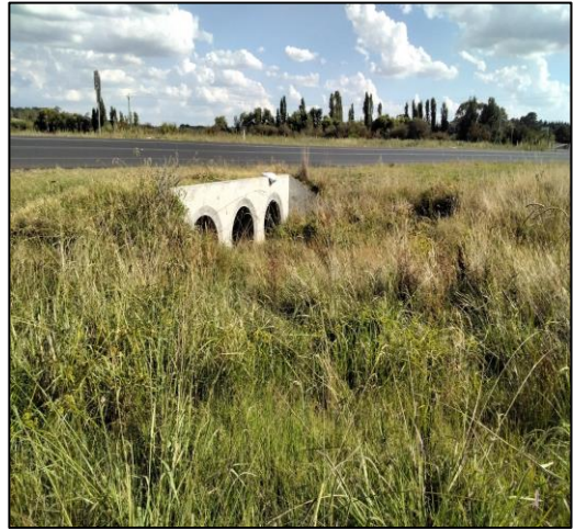
Photo 26 Culvert in Lot 200 facing southwest (30 January 2024)
