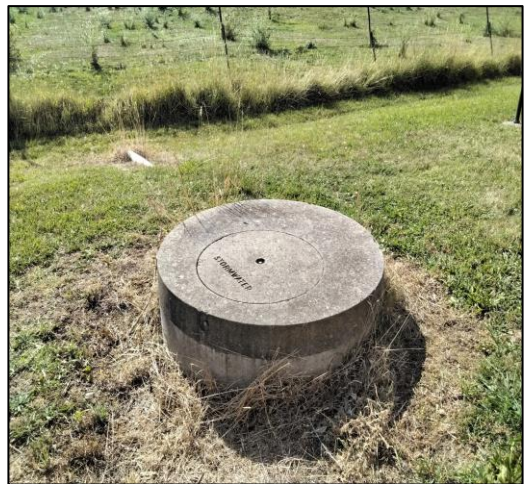
Photo 14 Stormwater drain within Lot 6 adjacent Lot 1 (30 January 2024)
