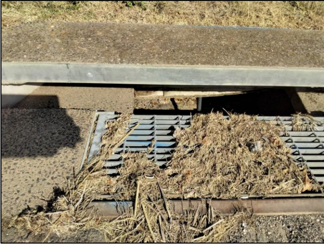
Photo 23 Stormwater drain (dry) within access road within Lot 6 (30 January 2024)
