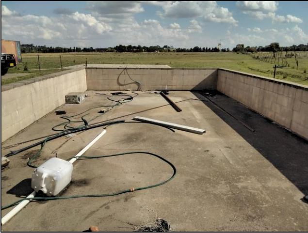
Photo 17 AST bund within Lot 6 facing south (30 January 2024)
