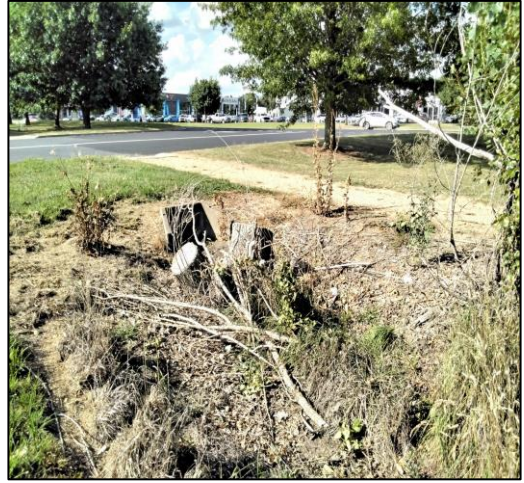
Photo 24 Culvert to the northeast within Lot 6 (30 January 2024)
