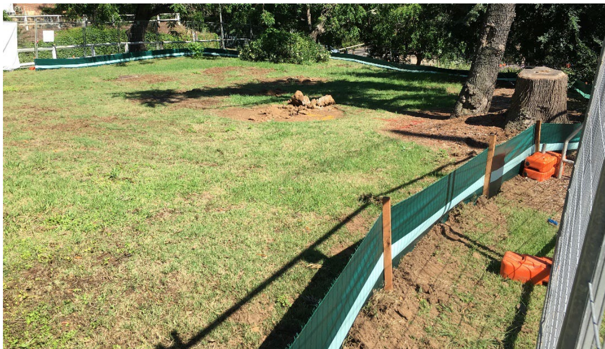
Figure 8. An appropriately installed sediment fence
