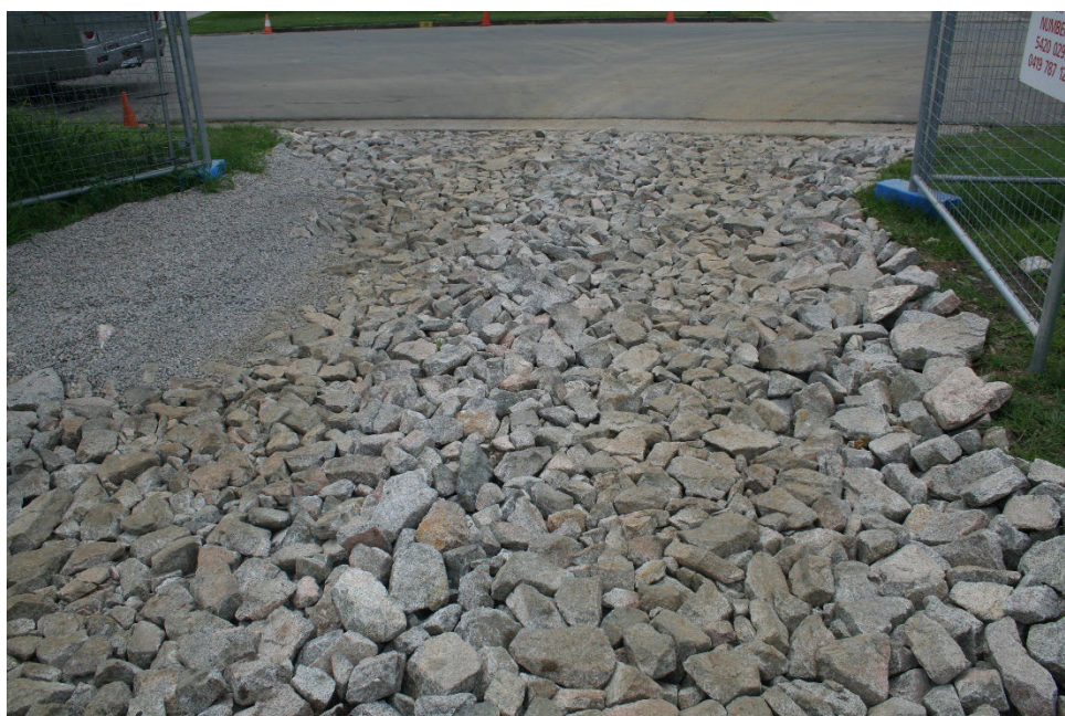
Figure 5. A stabilised site entry/exit point. Source: Catchments and Creeks Pty Ltd
