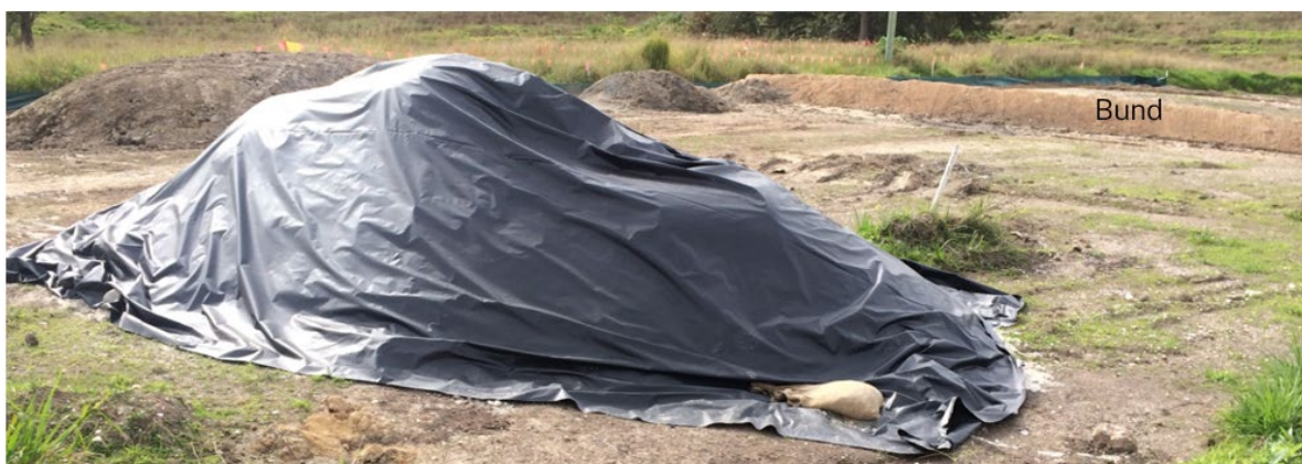
Figure 7. An unattended stockpile has been securely covered to prevent any loss of soil, with a compacted bund acting as sediment control downslope. Source: Department of Primary Industries and Regional Development – Fisheries
