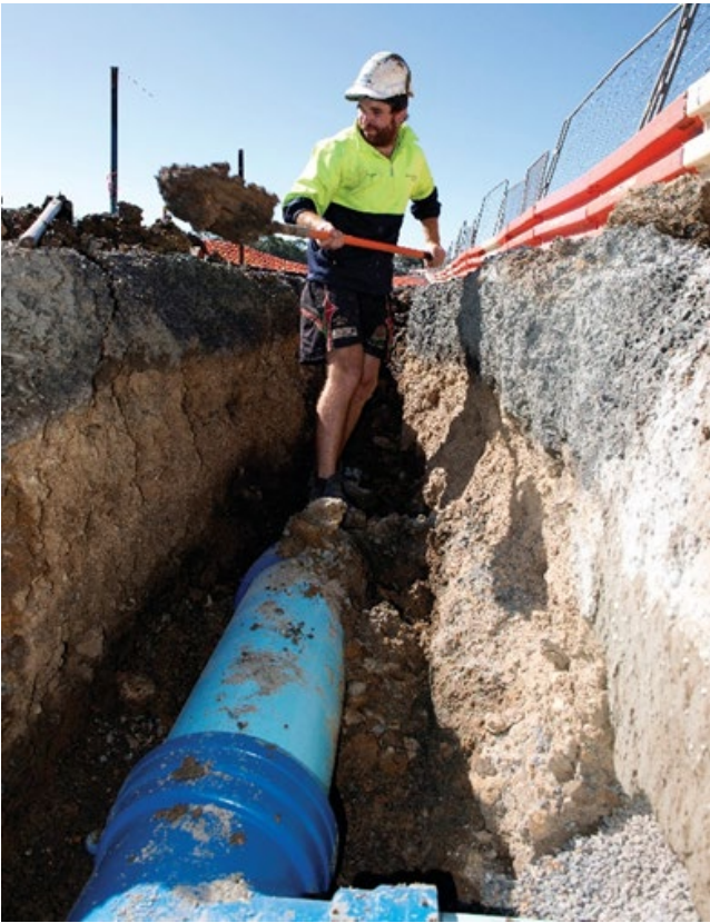
Figure 15. A construction worker installs a service trench
