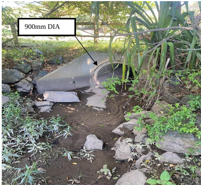
Figure 8: Headwall 1 located east to Jordan Esplanade toward south
