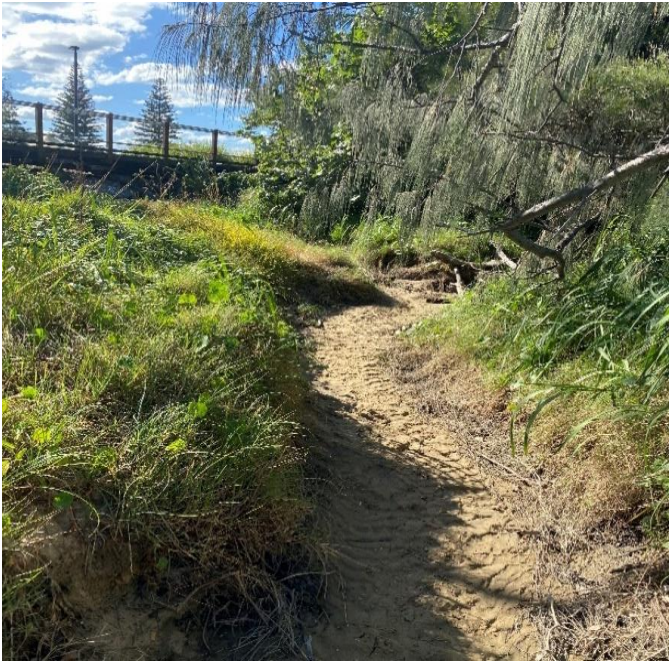
Figure 13: Swale collecting runoff from twin 250mm stormwater pipes (Outlet 3)
