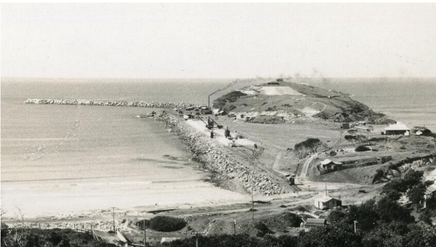
Figure 3.28: View facing east towards Corambirra Point from the mainland, showing completed retaining wall and area of reclamation, 1936. 58
