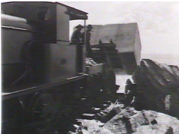
Figure 3.40: 40 tonne concrete block being placed at eastern breakwater, early 1930s. 76
