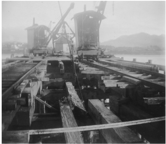
Figure 3.52: Construction of Coffs Harbour jetty extension, 1945 – showing timber girders being positioned. 93
