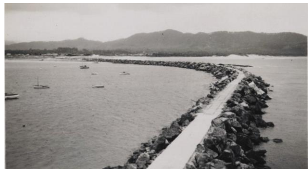
Figure 3.35: Northern breakwater from Muttonbird Island, ca. 1940s – showing concrete capping. 68
