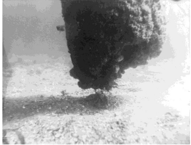
Figure 3.72: Department of Public Works dive inspections of Coffs Harbour jetty piles, 1975 – broken pile suspended above seabed, showing evidence of extreme marine borer damage. 124
