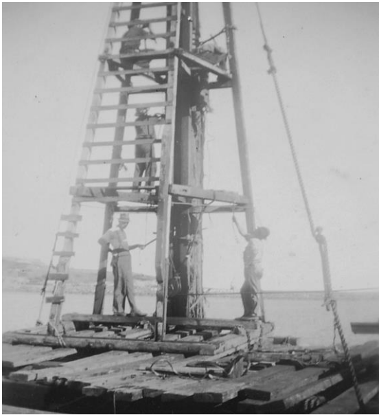
Figure 3.51: Construction of Coffs Harbour jetty extension, 1945 – showing close up of pile rig. 92
