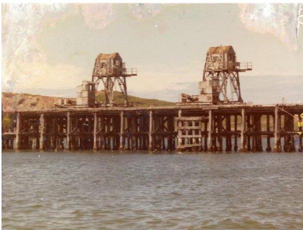
Figure 3.73: Stothert & Pitt cranes on Coffs Harbour jetty being disassembled, 1984. 125
