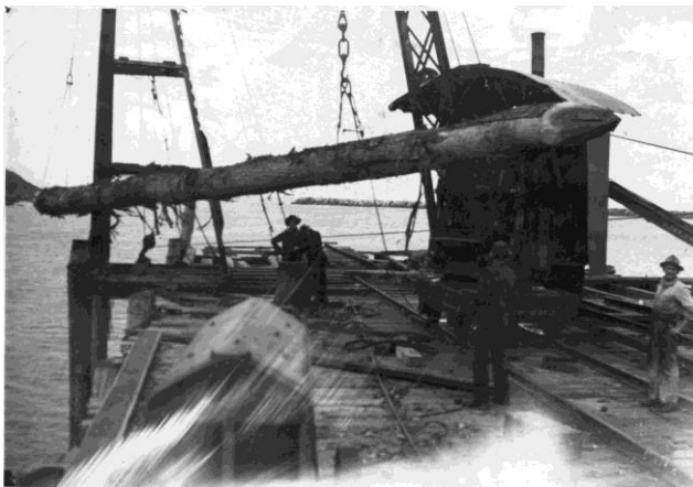
Figure 3.49: Construction of Coffs Harbour jetty extension, 1945 – showing timber pile being hoisted into position in pile driving rig. 90
