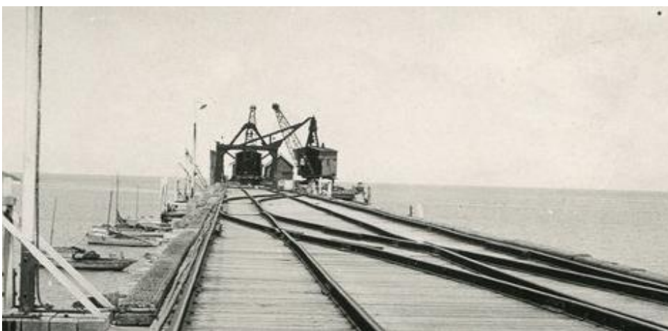
Figure 3.17: ca. 1930 view of Coffs Harbour jetty – showing widening and additional crane on southern side of jetty head. 37
