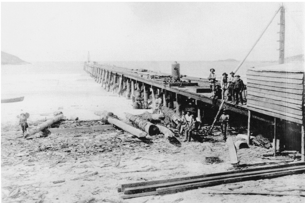
Figure 3.4: Construction of Coffs Harbour jetty, 1892 – pile driver in operation at the seaward end. 15
