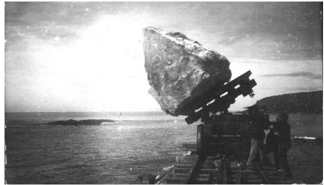
Figure 3.33: Construction of the northern breakwater; tipping rock from railway wagon ca. 1917. 66
