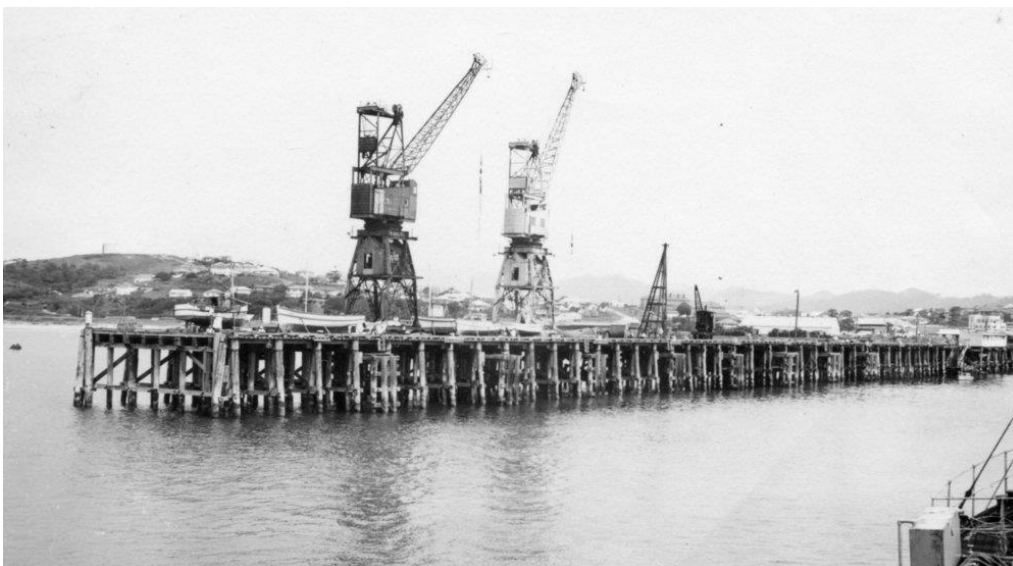
Figure 3.57: 1972 oblique aerial photograph of Coffs Harbour, showing extended and widened jetty with two Stothert & Pitt cranes. 101
