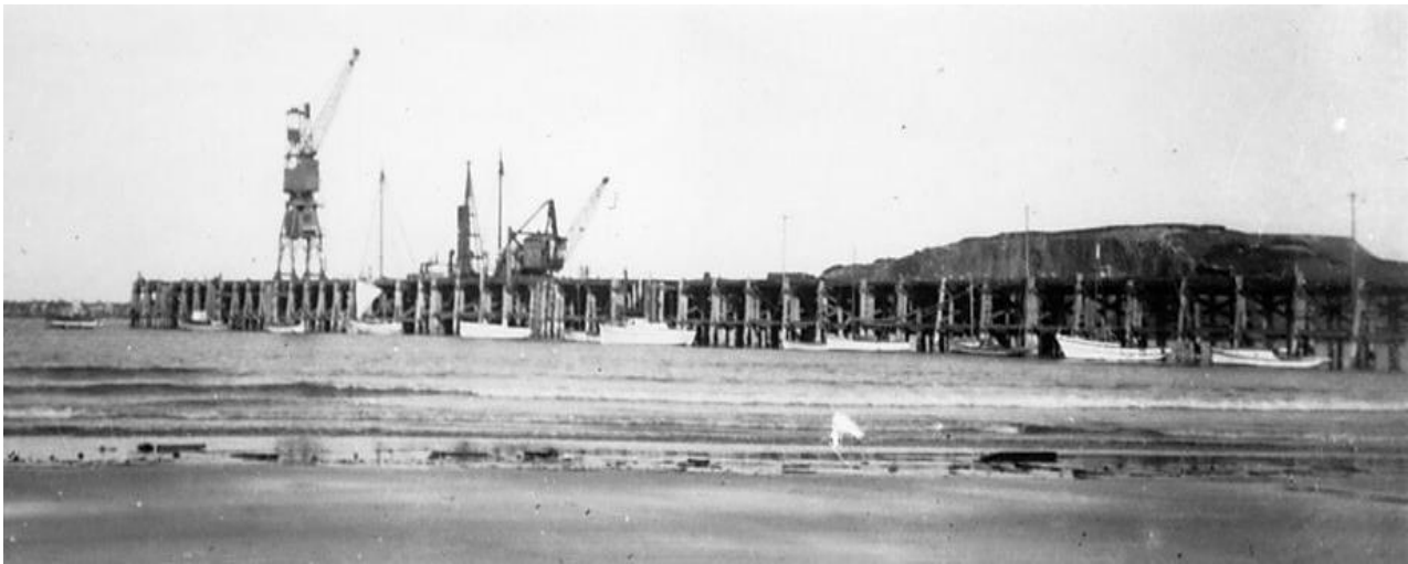
Figure 3.56: View of northern side of Coffs Harbour jetty, ca. 1952 – showing widening works in progress with pile driving rig adjacent to steam crane. 100
