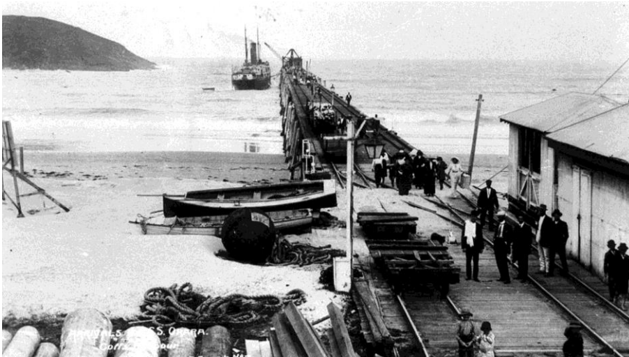
Figure 3.11: Coffs Harbour jetty ca. 1912 – showing duplicated rail lines and SS Orara unloading whilst moored off northern side of jetty. 28
