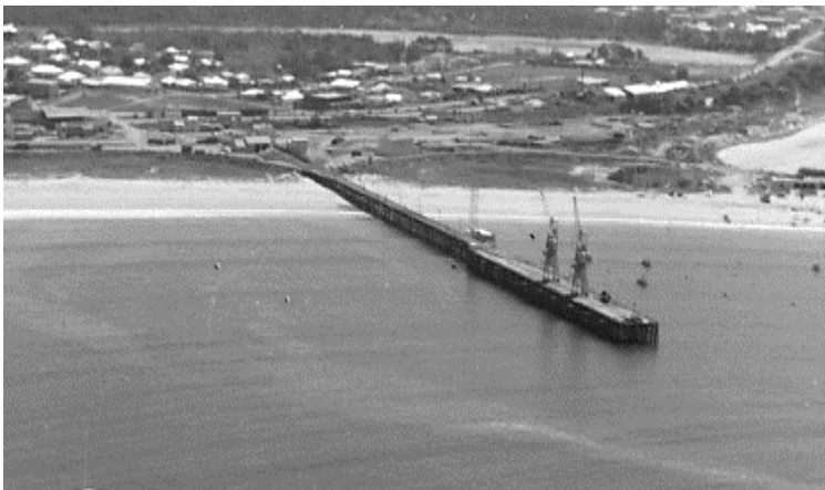
Figure 3.57: 1972 oblique aerial photograph of Coffs Harbour, showing extended and widened jetty with two Stothert & Pitt cranes. 101
