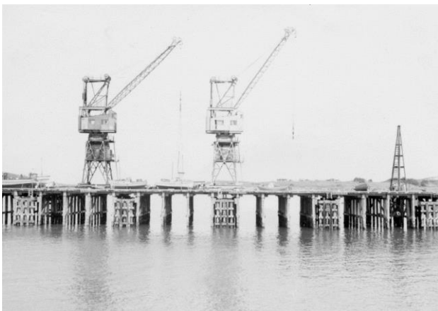
Figure 3.61: 1957 side view of Coffs Harbour jetty – showing strengthened sections for Stothert & Pitt cranes. 105
