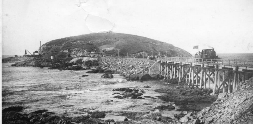
Figure 3.21: Timber trestle railway bridge between South Coffs Island and mainland, facing east with Corambirra Point quarry in background— showing Manning Wardle locomotive crossing the bridge, 1918. 50
