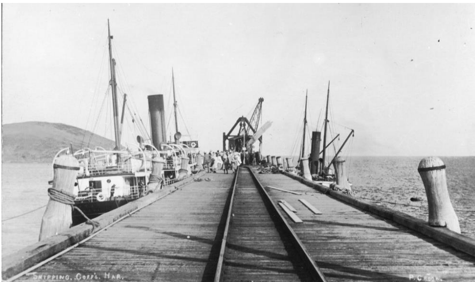
Figure 3.9: 1908 view of seaward end of Coffs Harbour jetty; showing original single tramway and 5 tone steam derrick crane. 23
