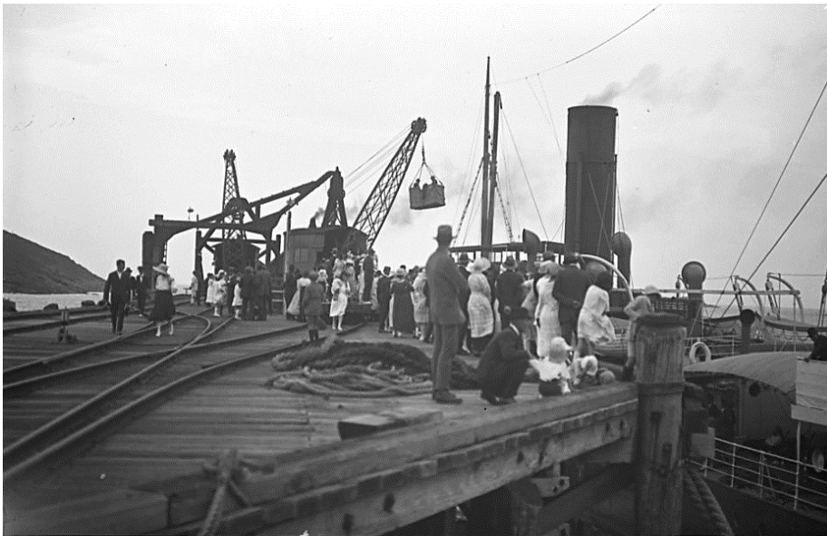
Figure 3.18: ca. 1920 view of passengers disembarking in the basket at Coffs Harbour jetty – showing widening on southern side of jetty head. 38
