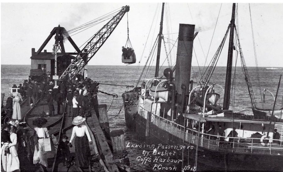
Figure 3.13: Landing passengers by basket from SS Cavanba at Coffs Harbour jetty. 30
