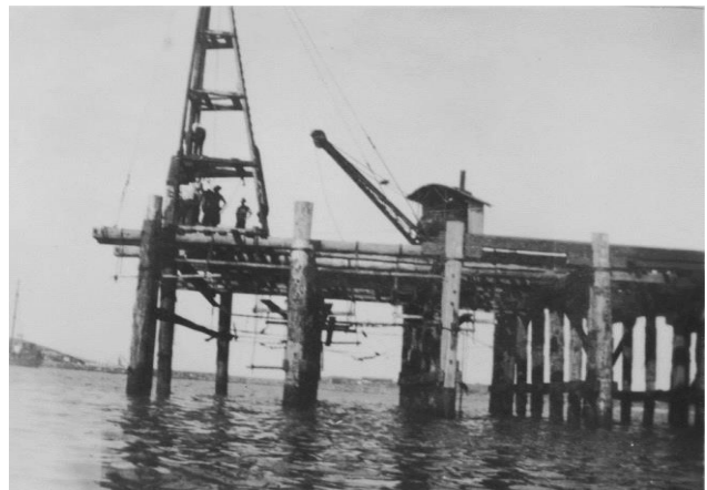
Figure 3.50: Construction of Coffs Harbour jetty extension, 1945 – showing timber pile being driven. 91
