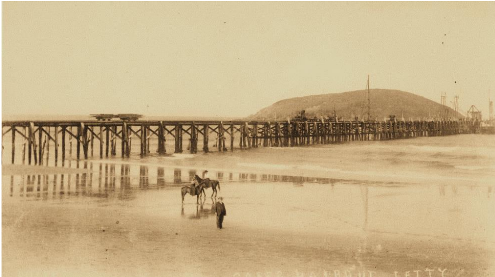
Figure 3.7: 1910 view of Coffs Harbour jetty facing north-west from beach; showing the three-pile trestle piers at landward end and five-pile trestle piers beyond low water mark. 21
