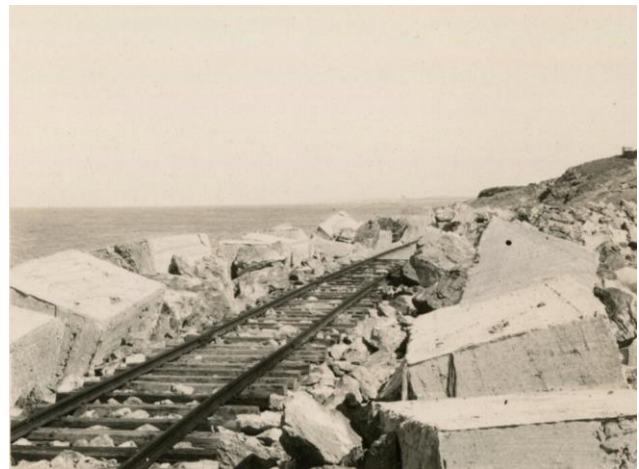
Figure 3.41: View towards end of the eastern breakwater, showing rock and concrete block placement, early 1930s. 77
