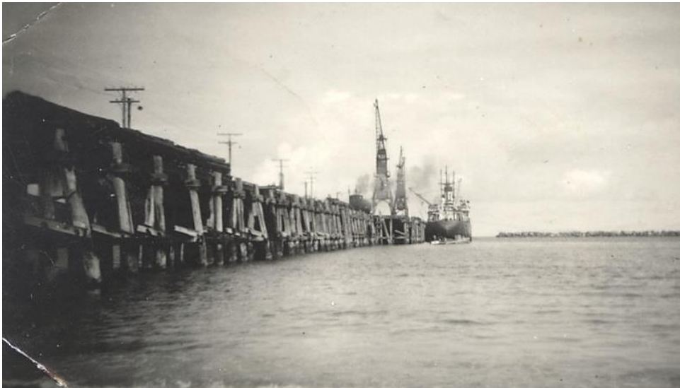
Figure 3.60: ca. late 1950s view of southern side of Coffs Harbour jetty – showing widened seaward end, with cargo vessel being loaded by Stothert & Pitt crane. 104
