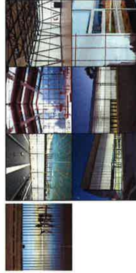
3. TRANSLUCENT FACED PANEL GLAZING - DANPALON ALUMINUM FINISHING - WHITE BLACK
