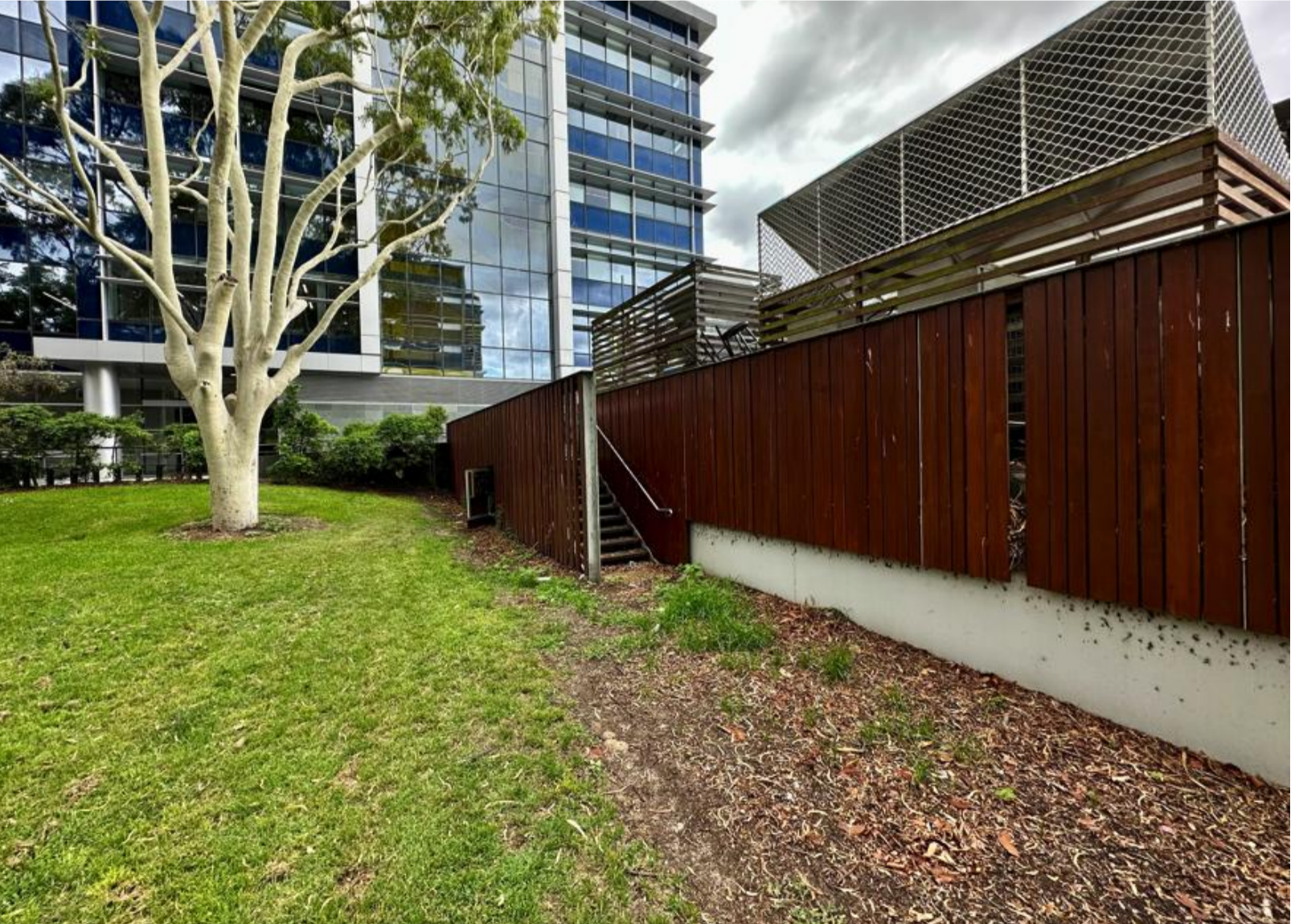
View from Stockroute park. Timber cladding to balustrade in need of upgrade.
