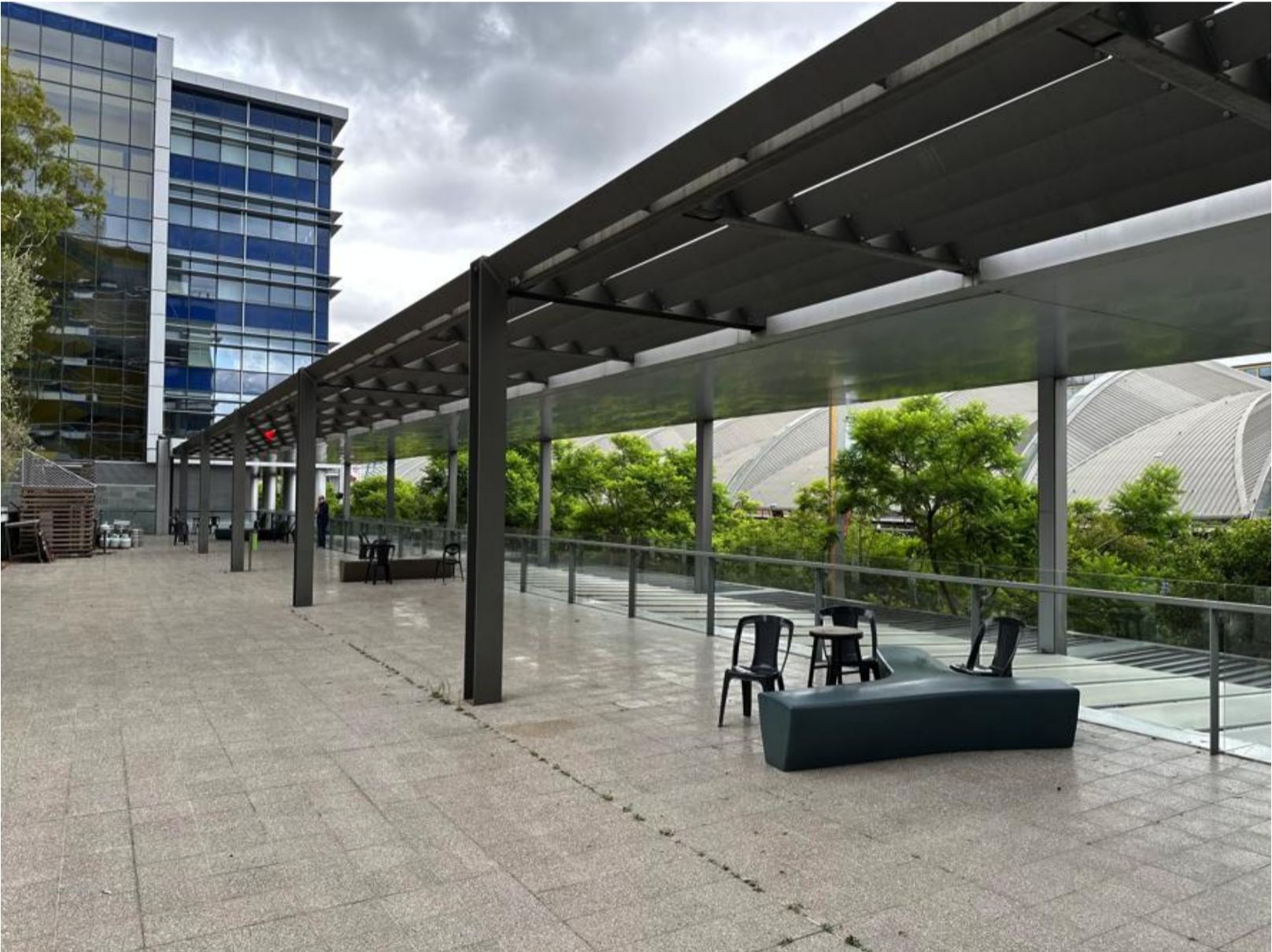
Existing steel structure with open louvres above.
