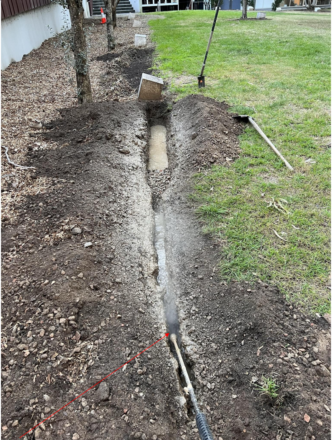
Image m: Hydro Excavation
