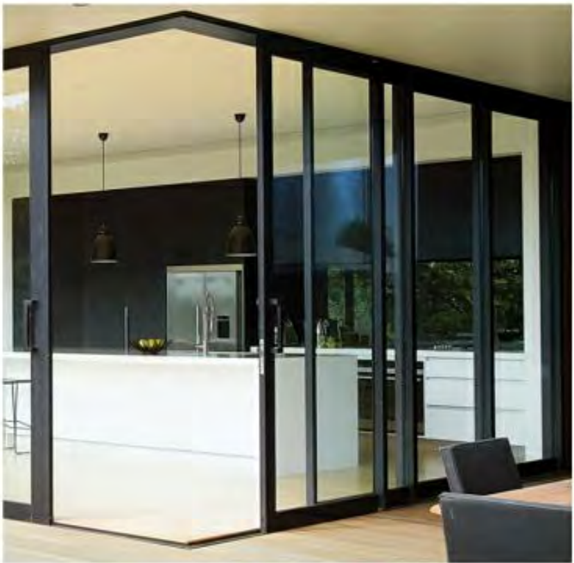
GL1: FIXED GLAZING WITH OPERABLE DOORS Clear
