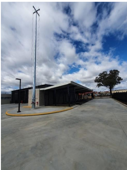
Figure 6 Fire hose drying pole
