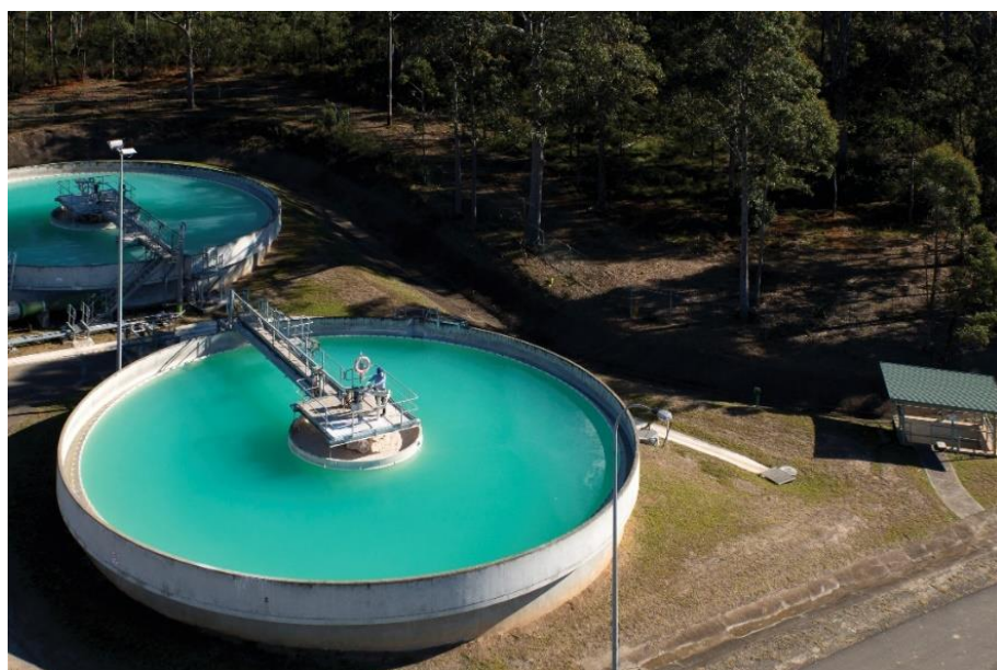
Figure 8 Basin at Prospect Water Treatment Plant
