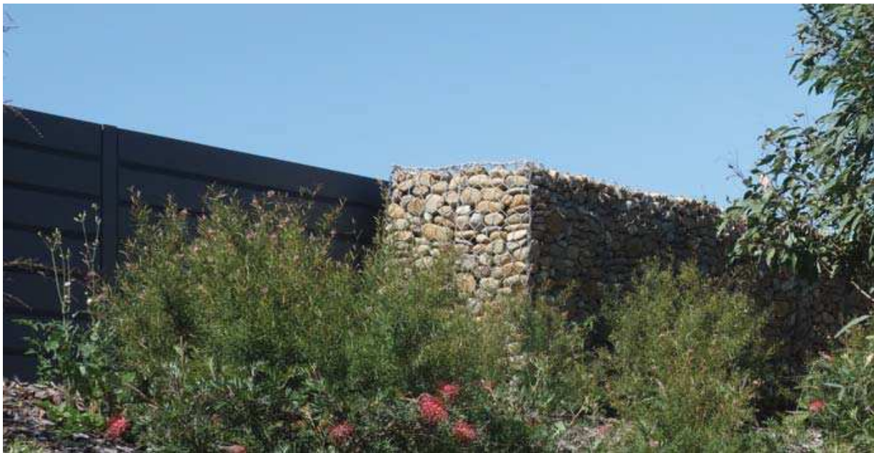
Figure 2-17: Indicative rock gabion and timber acoustic wall.
