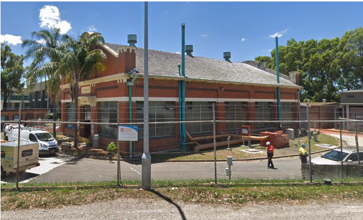
Figure 8 SP0067 Sydney Water Pump Station
