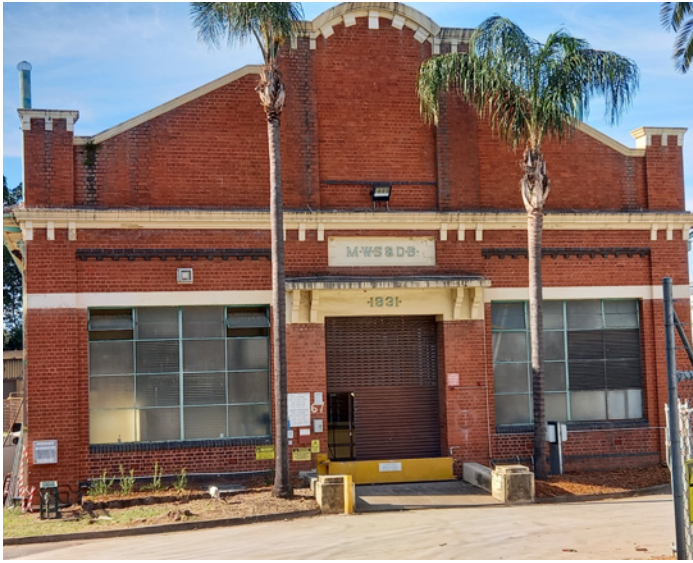
Sewage Pumping Station 67 front facade
