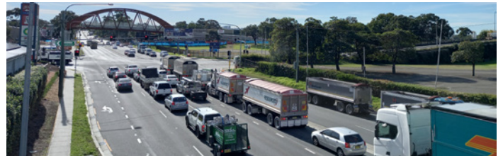
The Parramatta Light Rail bridge over James Ruse Drive looking north east
