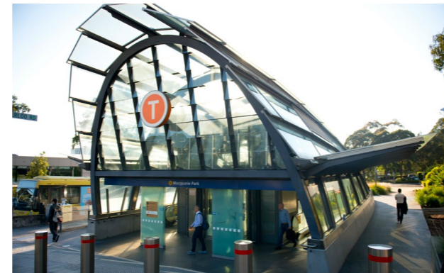
Macquarie Park Metro Station
