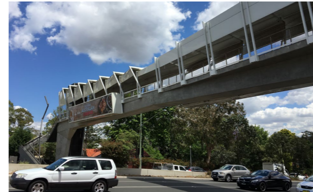
Pedestrian Bridge over Epping Road
