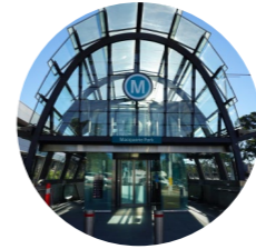
Metro station upgrades and increased connectivity
