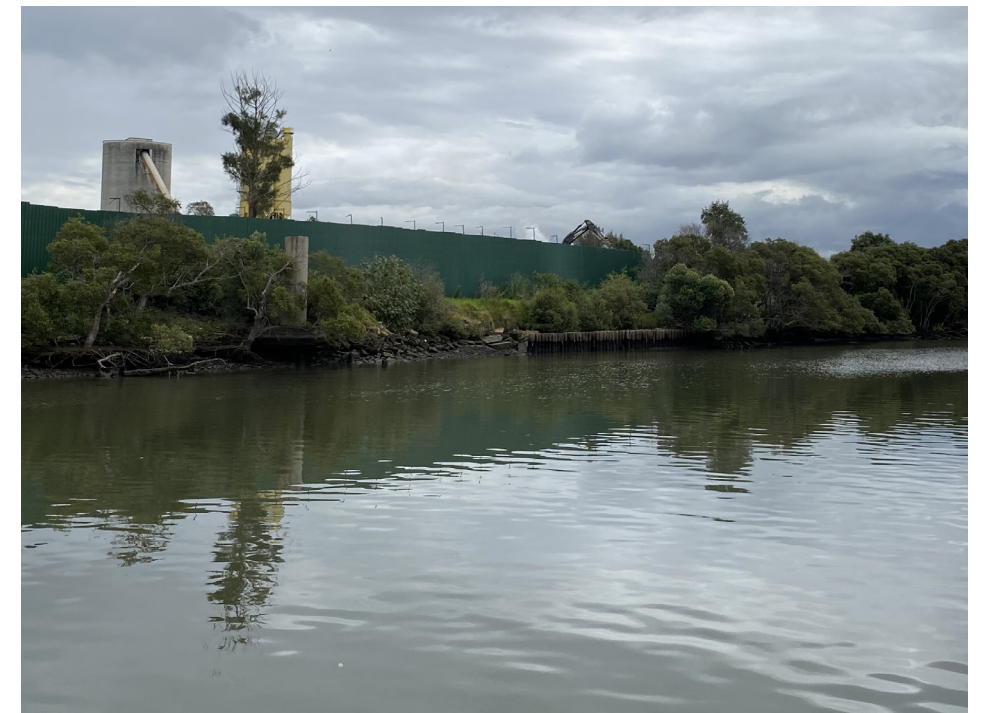
15. Remnants of Industrial Wharves at Camellia.
