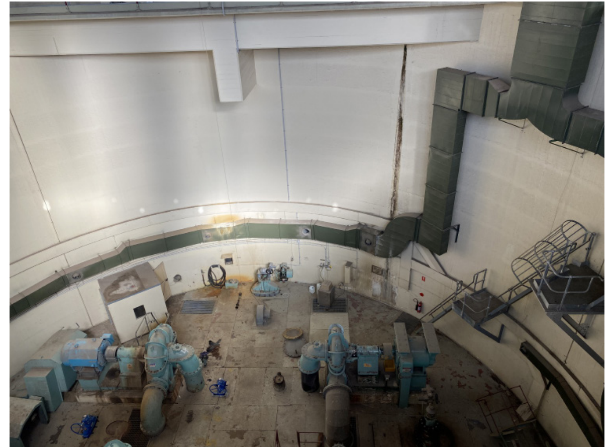
1. Pumping Station 67 subfloor area.
