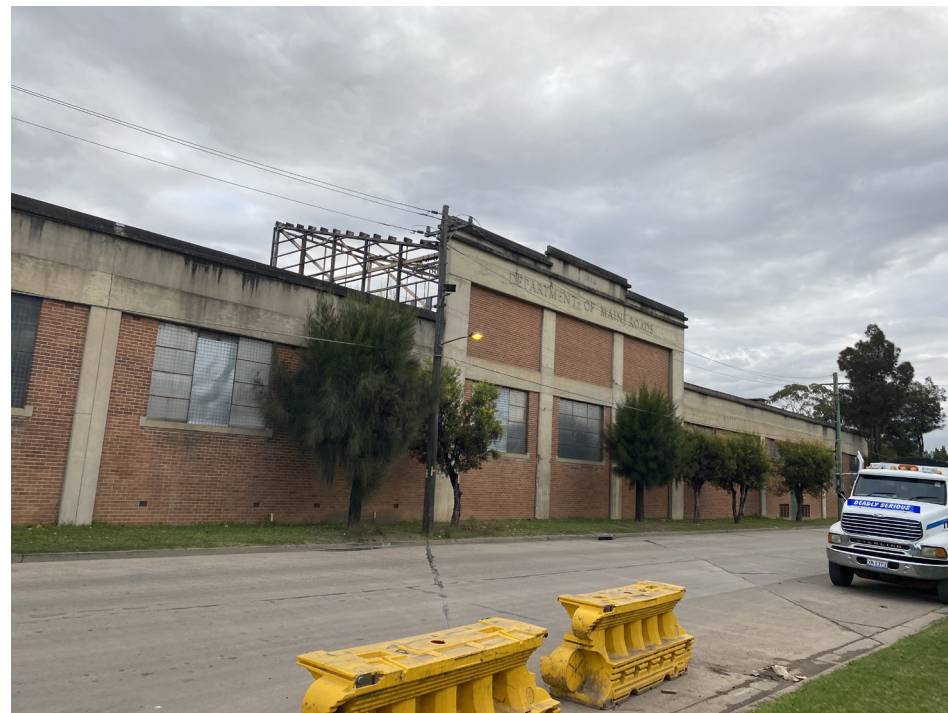
13. Department of Main Roads former workshop and depot, 1944.
