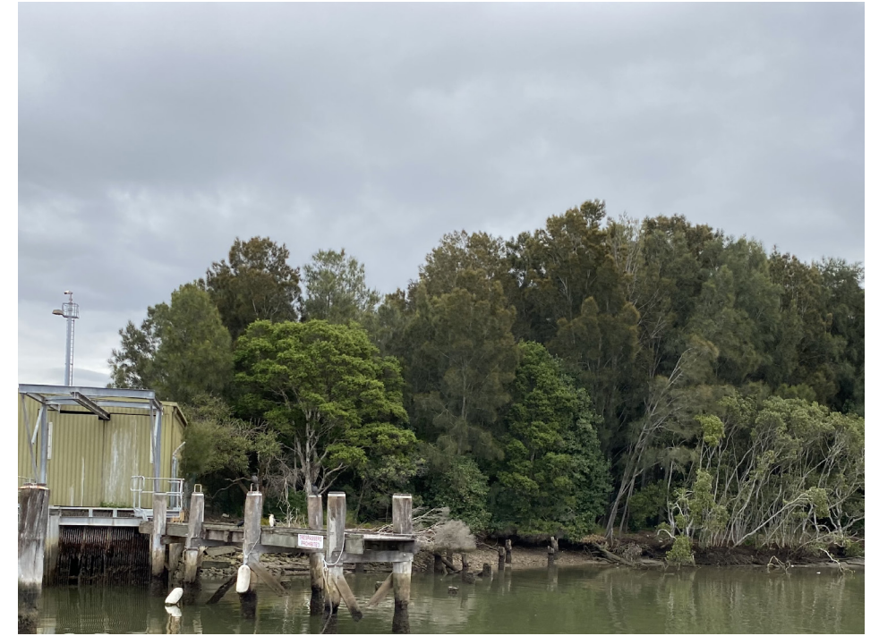
14. Shell Oil Refinery wharf and remnant structures.
