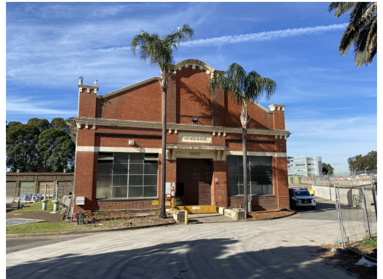
2. Pumping Station 67 front facade.
